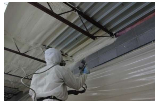
Sealing Roof-Wall Gap
