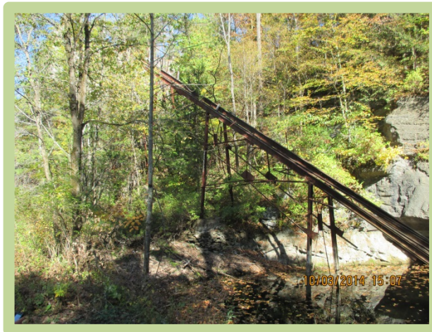
Abandoned mining facilities on the Snyder Mine Property
