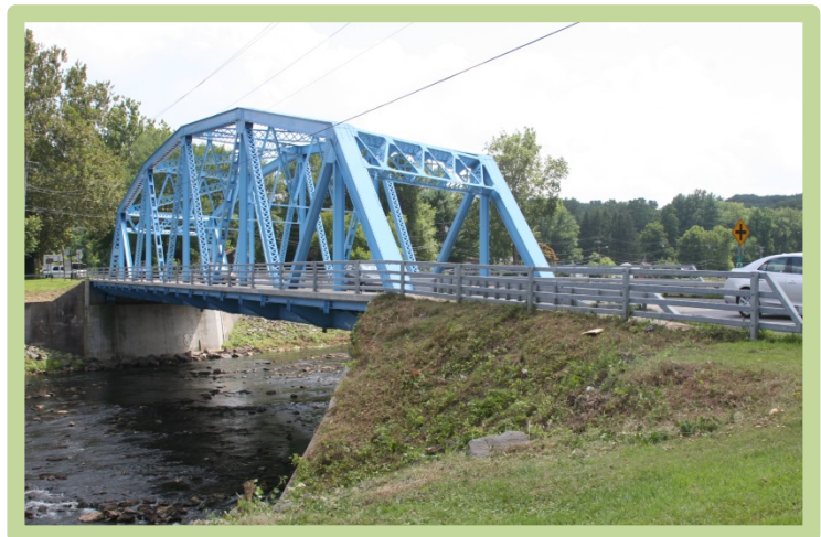
Rondout Creek Bridge looking south down Route 32
