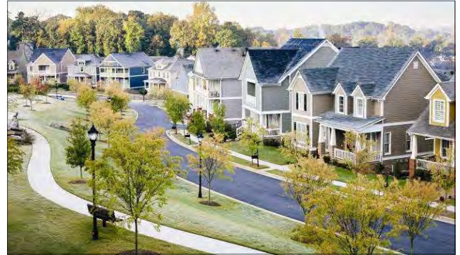
Sidewalks in new developments can improve safety, mobility, and convenience for all users.
