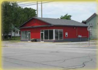
Former Alaskan Oil/Marino's
