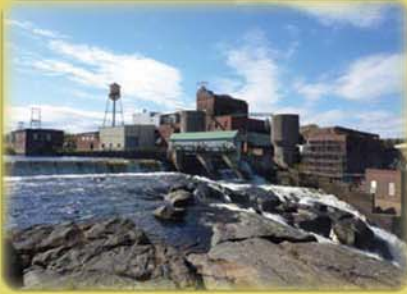
Former Lyons Falls Paper Mill *A North Country Regional Council Transformational Project*
