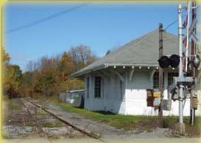
Train Station / Agway Property
