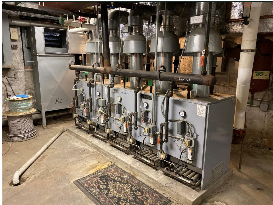
Photo 2-5. 1,500,000 Btu/Hour Hydro Therm MR-1500B
