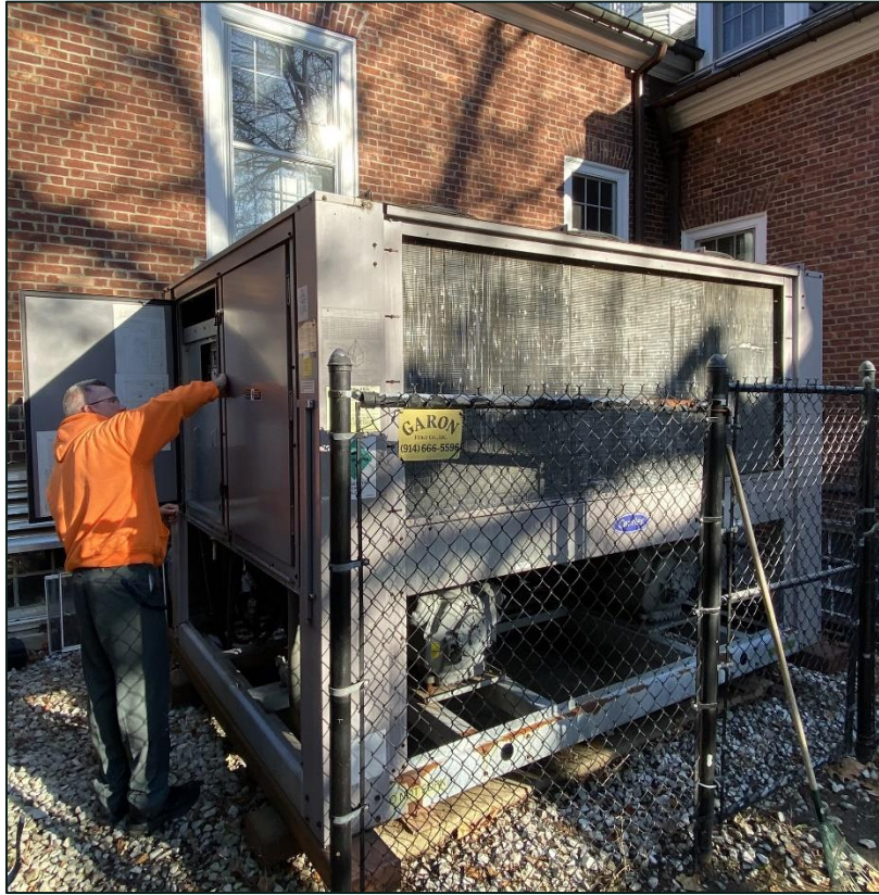
Photo 2-4. 60-Ton Carrier 30GTN060
