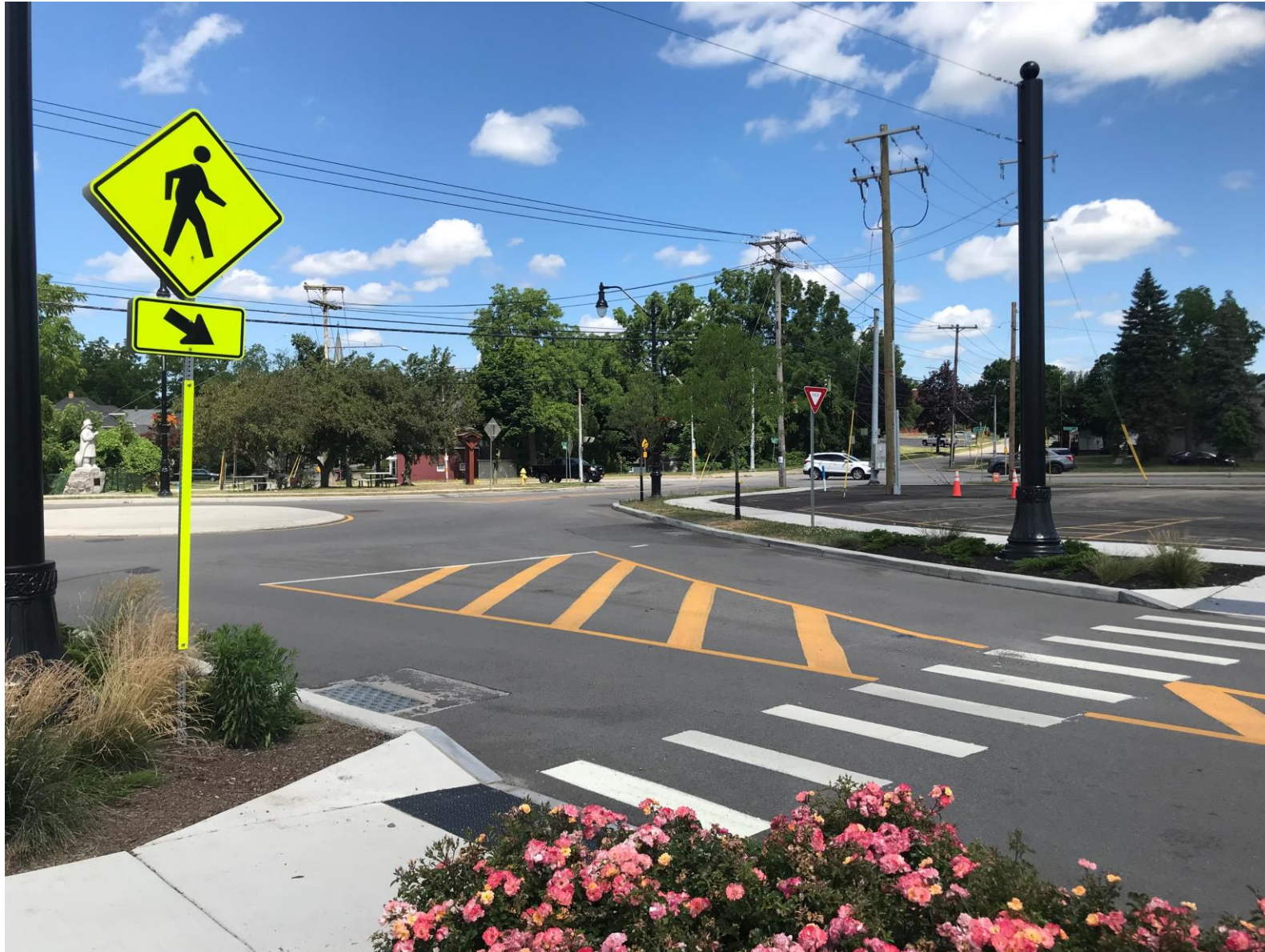
Marked crosswalk and pedestrian signage at the new roundabout at the intersection of West Main Street and Aurora Avenue
