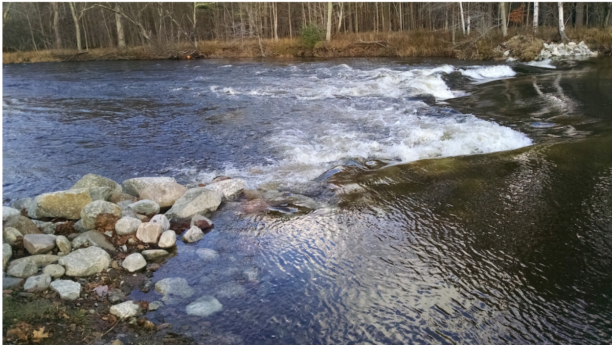
Figure 6. A W-weir installed in the Town of Keene on the East Branch of the Ausable River in 2015 replaced an old wooden recreational dam. Upstream (right) the weir protects a swimming hole. Downstream roughness creates fish habitat for native trout. Photo taken immediately after bankfull event.
