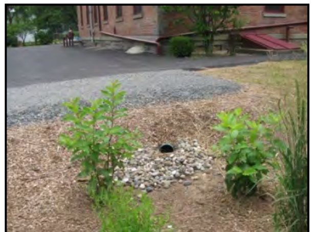
Example of a rain garden and stormwater drainage at the Kingston Library. (Source: NYS DEC)
