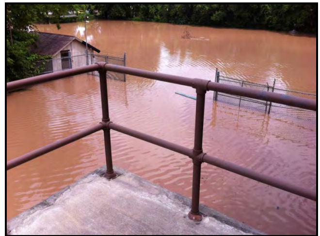
Flooding at Oneida Armory (Source: City of Oneida)
