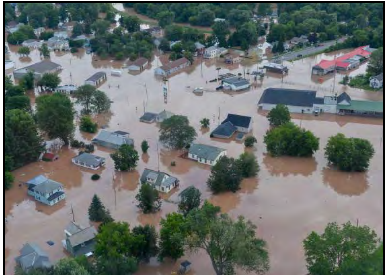
Storm Damage (Source: Madison County)
