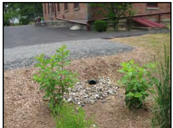
Example of a rain garden and stormwater drainage at the Kingston Library. (Source: NYS DEC)
