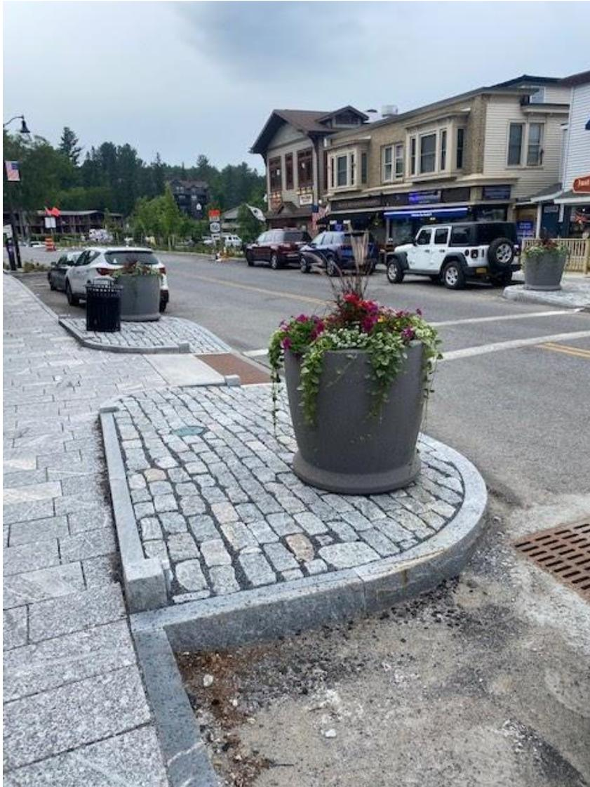
Photo 4: New crosswalk with bump out and planting to increase pedestrian visibility and safety
