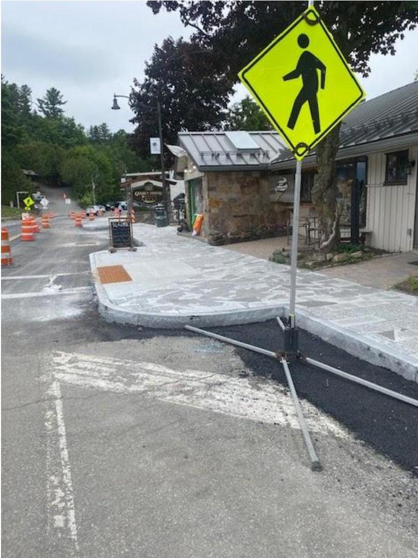
Photo 5: New crosswalk with bump out on the South End of Main Street to improve pedestrian visibility and safety
