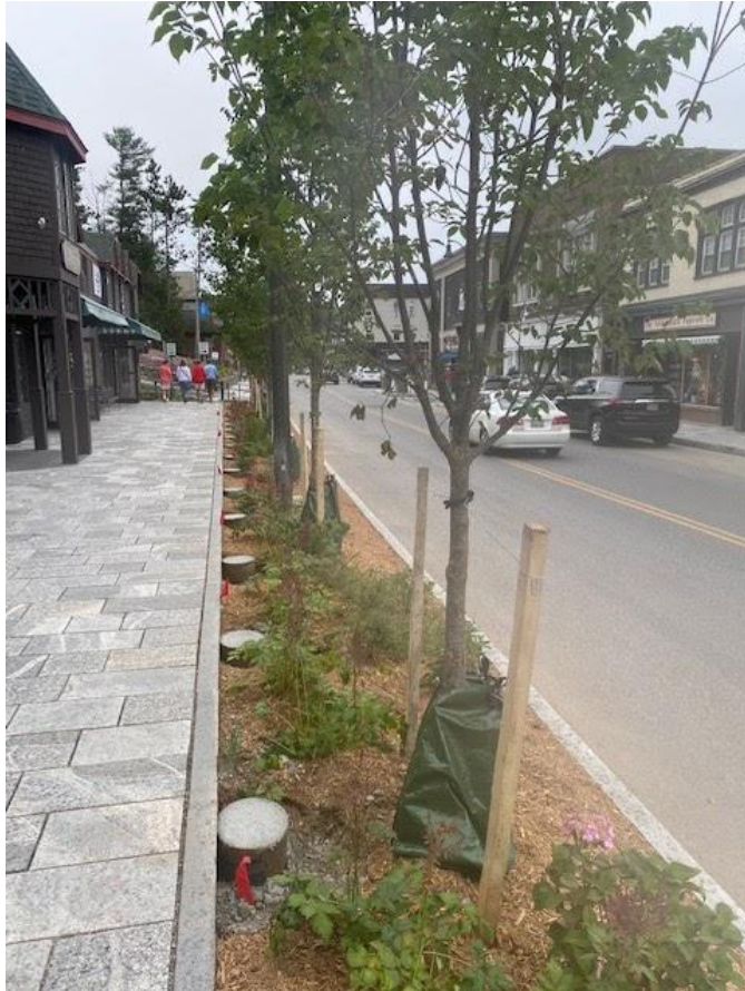
Photo 1: Street trees planted in front of 2464 Main Street, Lake Placid
