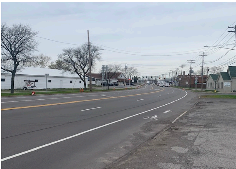
Image three shows the added bike lanes and car lane reduction from 4 to 3. Take at River Road nearing intersection with Main Street
