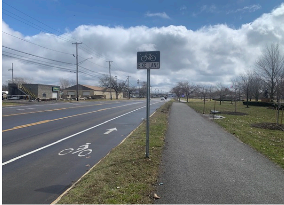
Image One: shows new River Trail bike lane, repaved old trail (now walking trail). Taken at Veteran's Park on River Road
