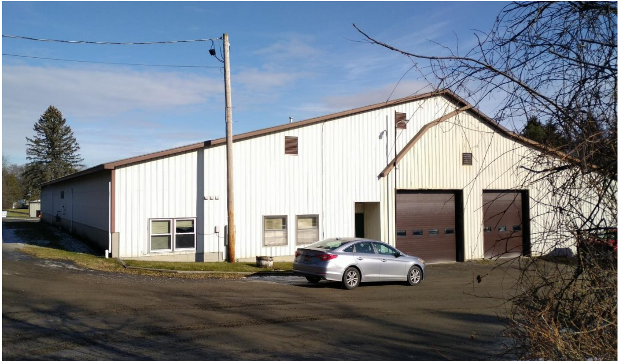
Photo: Newfield Town Barn - the roof profile of the original barn can be seen directly above the double doors. The 1976 addition is obscured by the later 1993 addition to the left of the original barn.
