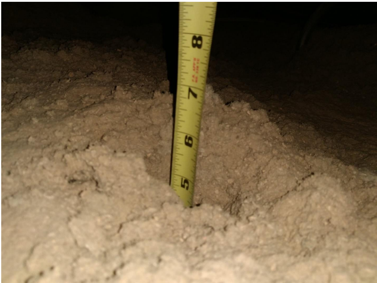
Photo: The attic is insulated with approximately 5.5 inches of loose cellulose.
