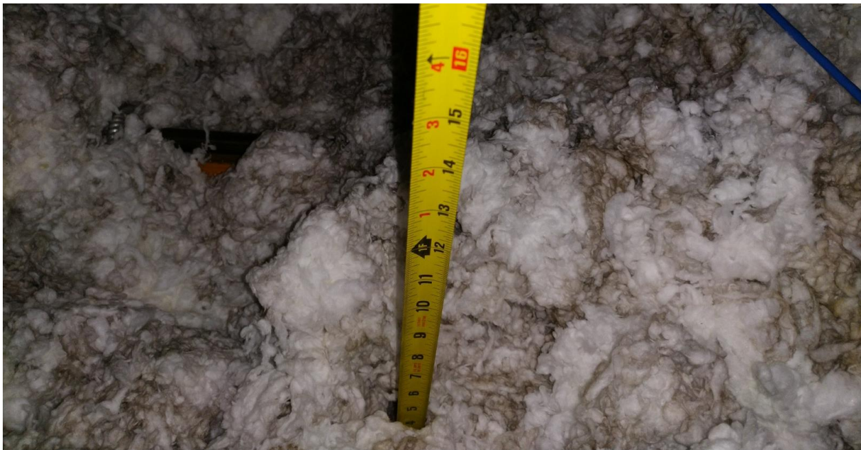
Photo: The attic is insulated with approximately 8 inches of loose fiberglass.
