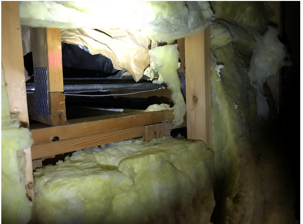
Figure 2, section of missing insulation
