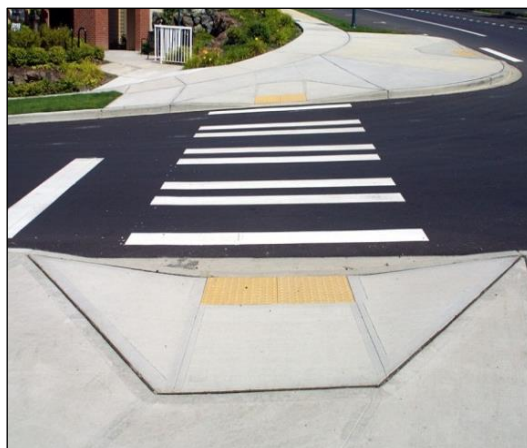
Figure 14: Curb Ramp
