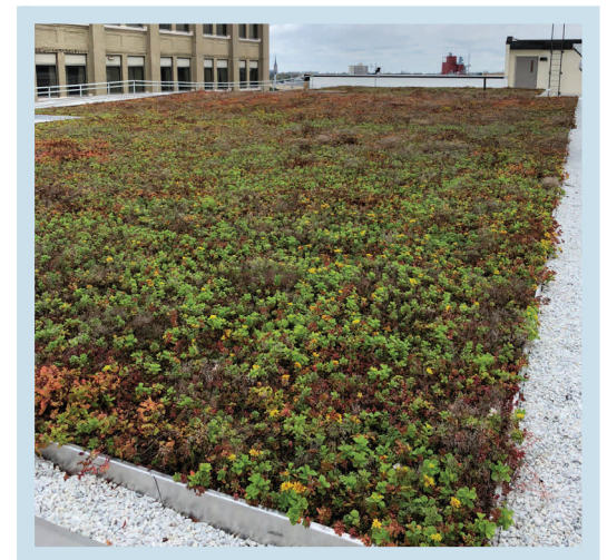
Figure 3. Roof of building 3 after construction of the green roof.
