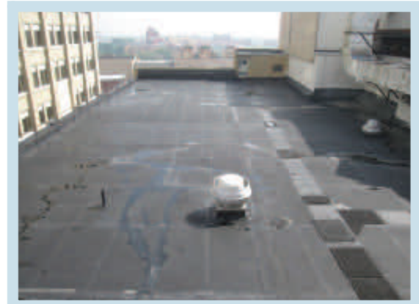
Figure 2. Roof of building 3 prior to the construction of the green roof.
