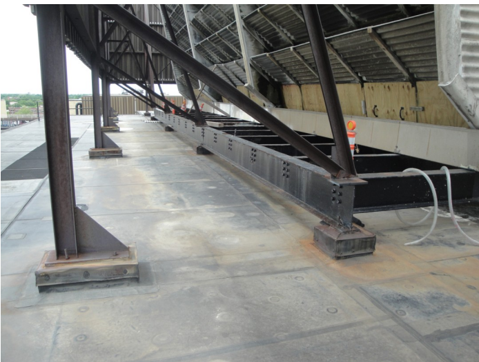
Figure D.14: Building 16—Detail view of cooling tower frame
