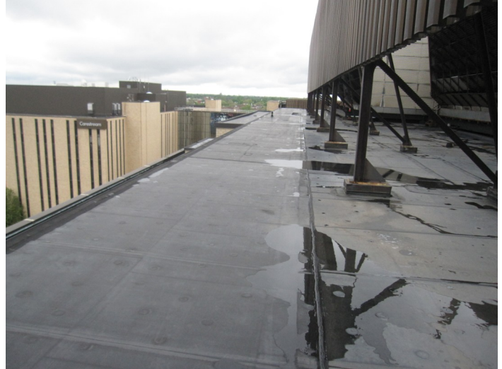
Figure D.9: Building 16—Overall view of roof, looking north
