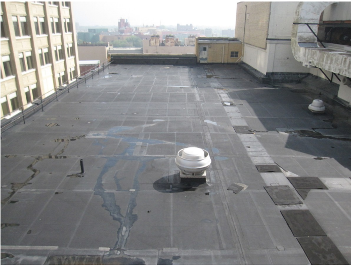
Figure D.1: Building 3—Overall view from above, looking east
