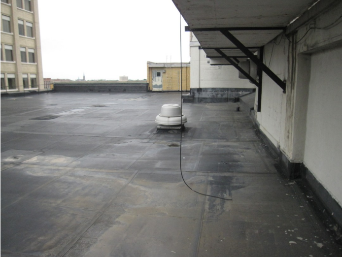
Figure D.5: Building 3—View of roof from entrance, looking east
