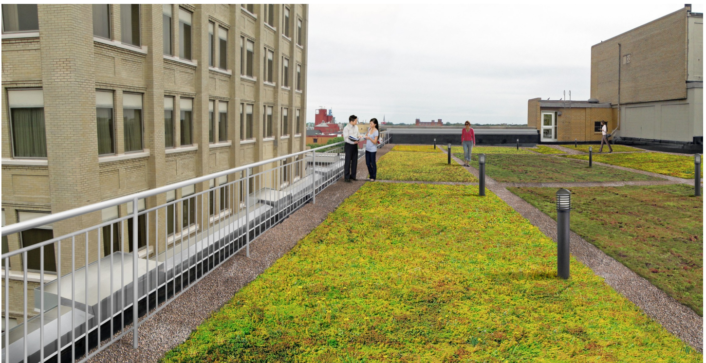
Figure D.18: Building 3. View of roof, looking north east, showing conceptual layout of proposed vegetated roof. Enhancements such as guard-rail, lighted bollards, and exit door into stair tower provided in consideration of public roof access.
