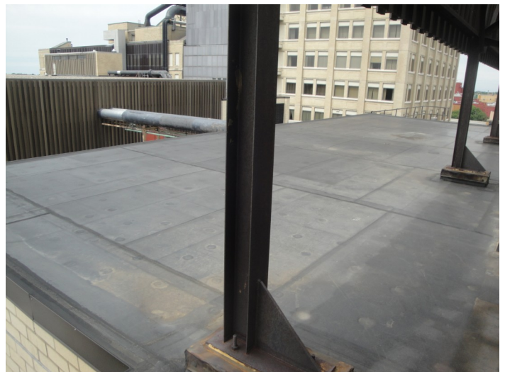
Figure D.15: Building 16—View of northern end of roof, looking north
