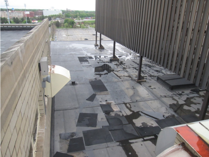
Figure D.8: Building 16—Overhead view of roof near entrance, looking west
