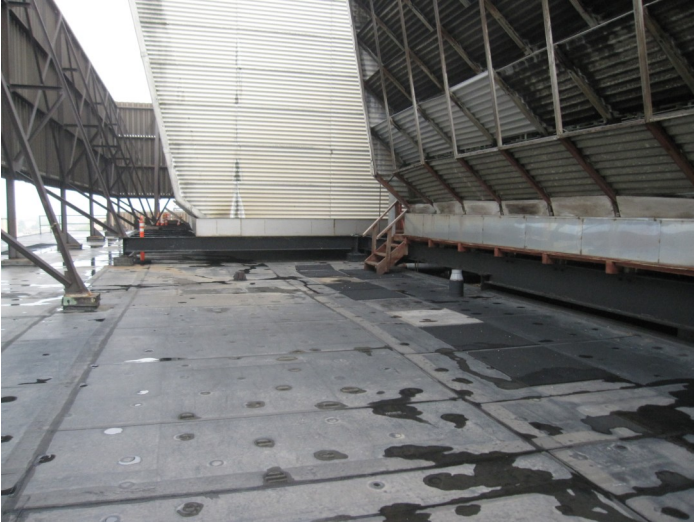
Figure D.12: Building 16—View of cooling towers at interior roof edge
