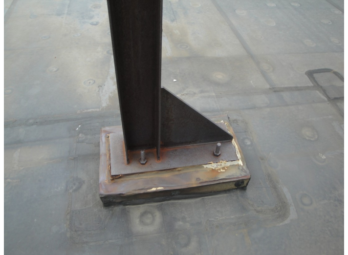
Figure D.13: Building 16—Detail view of equipment screen support
