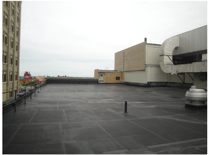
Figure D.2: Building 3—Overall from roof level, looking east
