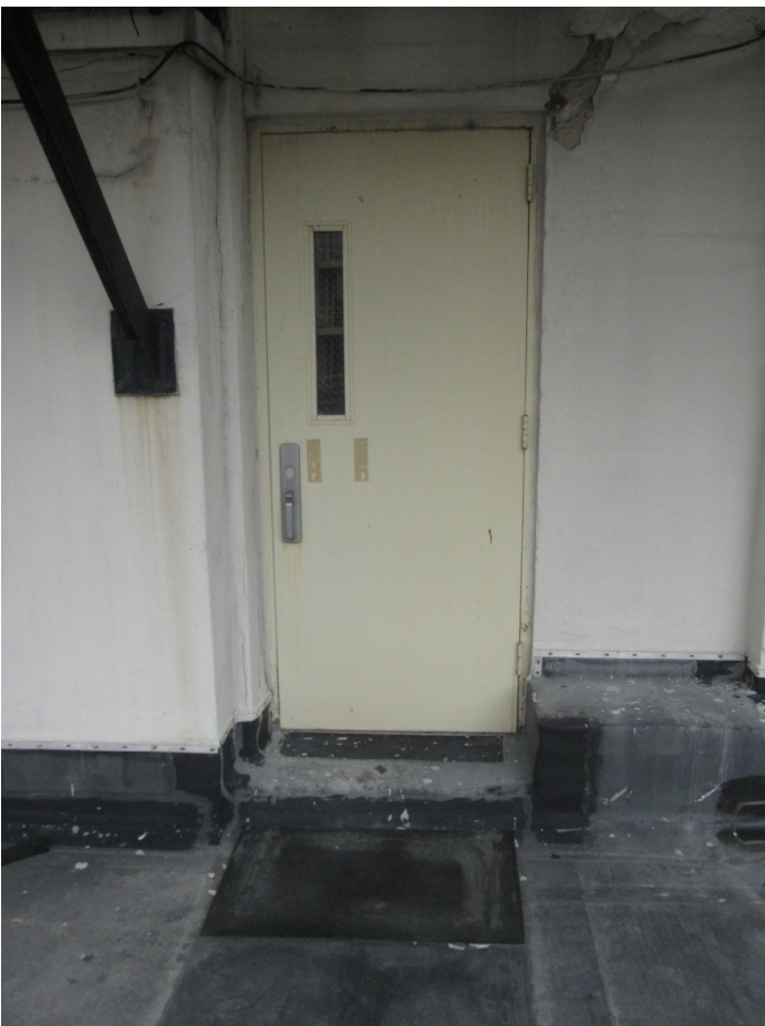
Figure D.7: Building 3—View of entrance door from exterior
