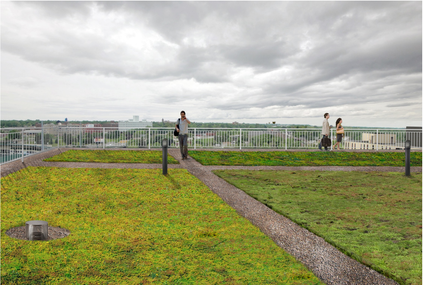
Figure D.20: Building 16. View of roof, looking south west, showing conceptual layout of proposed vegetated roof. Enhancements such as guardrail and lighted bollards provided in consideration of public roof access.
