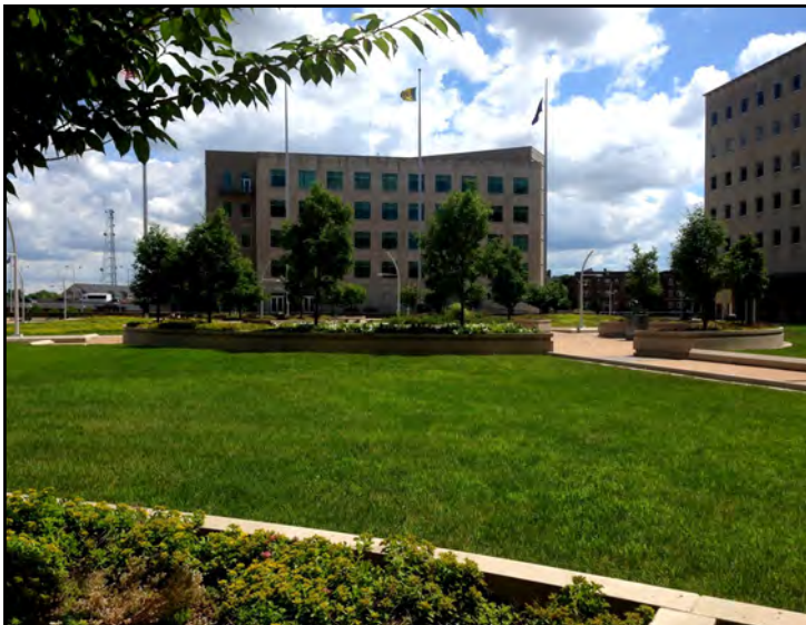
Monroe County Civic Center (below)
