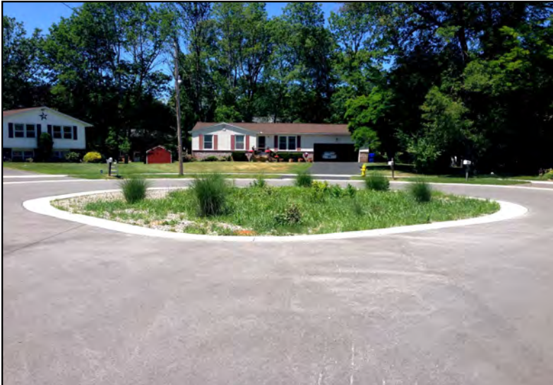
Cul-de-sac reduction retrofit with bioretention
