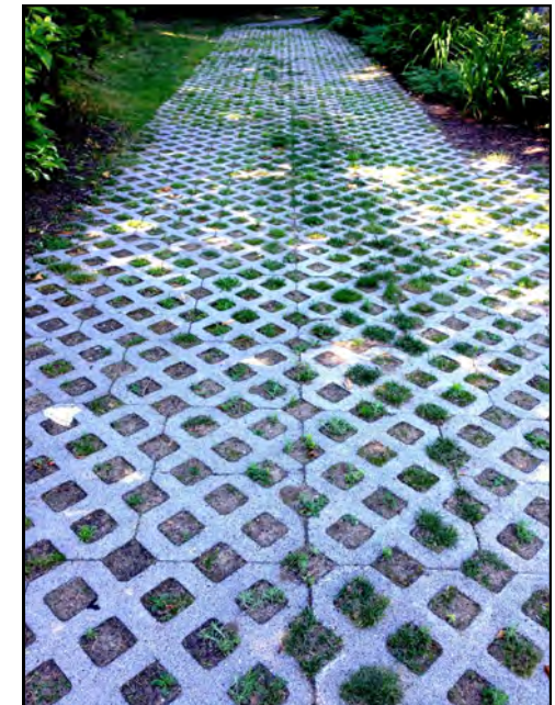
Permeable/grass pavers ( below )
