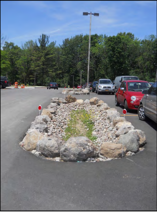
14 BIO-RETENTION ISLAND NOTE: BIO-RETENTION ISLANDS ARE TO BE EXCAVATED AND BACKFILLED FOLLOWING RESTORATION AND PAVEMENT SUBBASE INSTALLATION.
