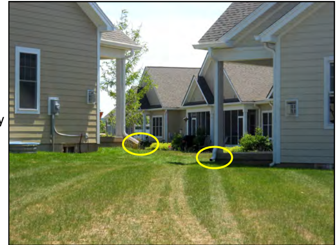
Rooftop disconnection ( above )
