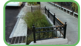
Elmwood Avenue stormwater planters installed.
