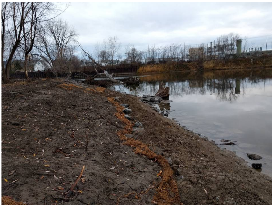
Photo 17. Reach 3. Looking downstream. 30 November 2016. Toe protection and rootwads shown near river edge.
