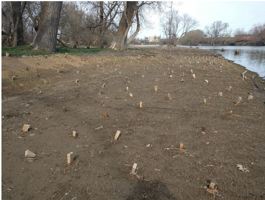
Photo 4. Reach 1 Looking Downstream; 13 April 2017. Sedimentation apparent on floodplain bench.
