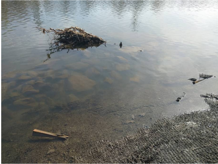
Photo 5. Reach 1. Stone toe protection and rootwad.
