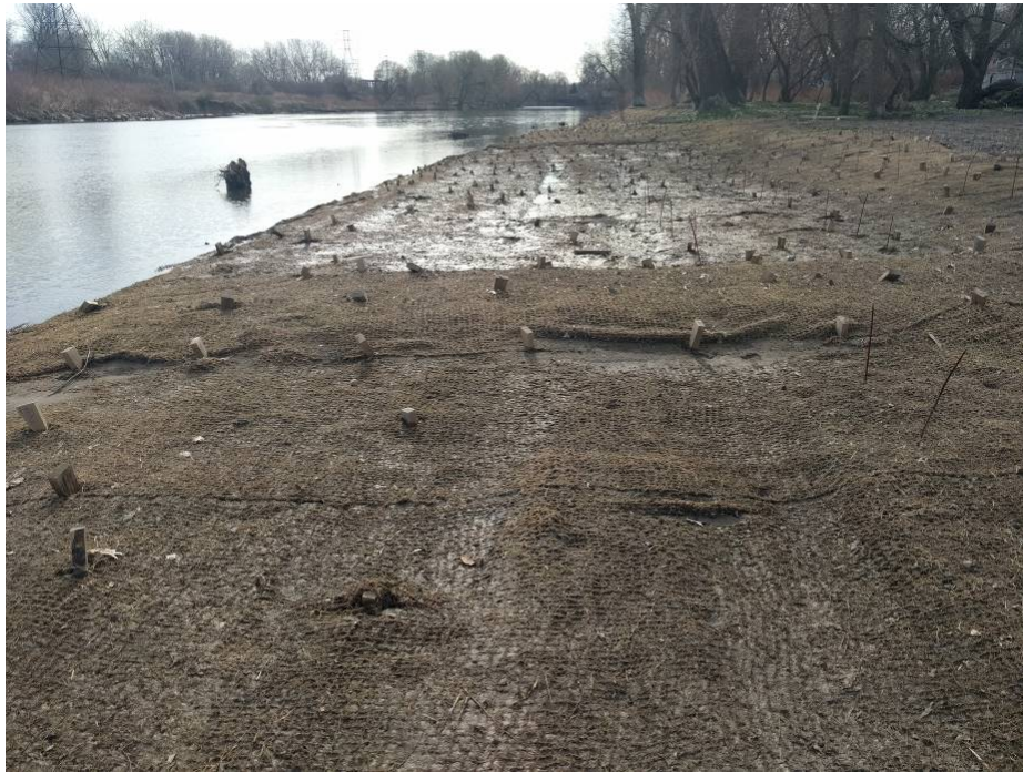
Photo 3. Reach 1 Looking Upstream; 13 April 2017. Initial indications of sedimentation on floodplain bench.
