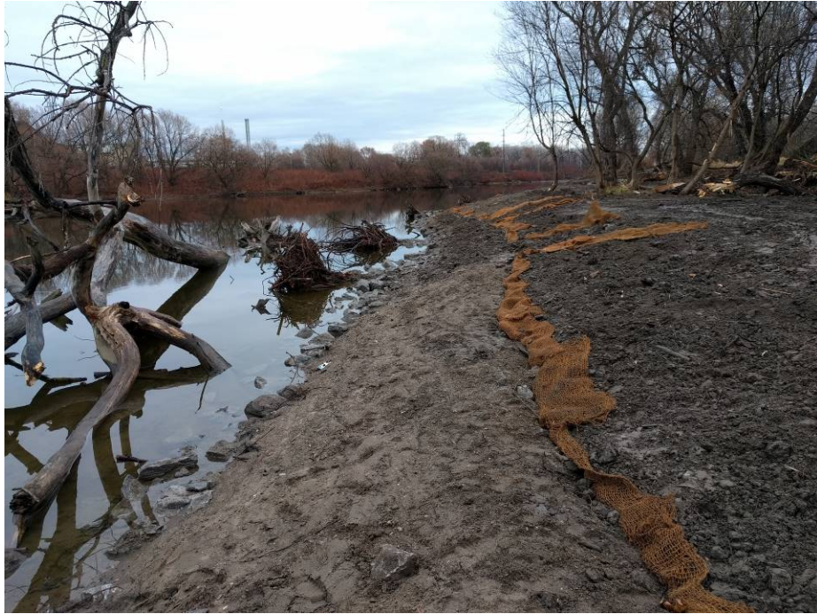
Photo 18. Reach 3. Looking upstream; 30 November 2016. Toe protection and rootwads shown near river edge.
