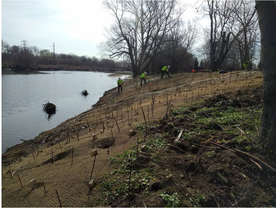
Photo 20. Reach 3a. Looking upstream; 13 April 2017. Live stake installation.
