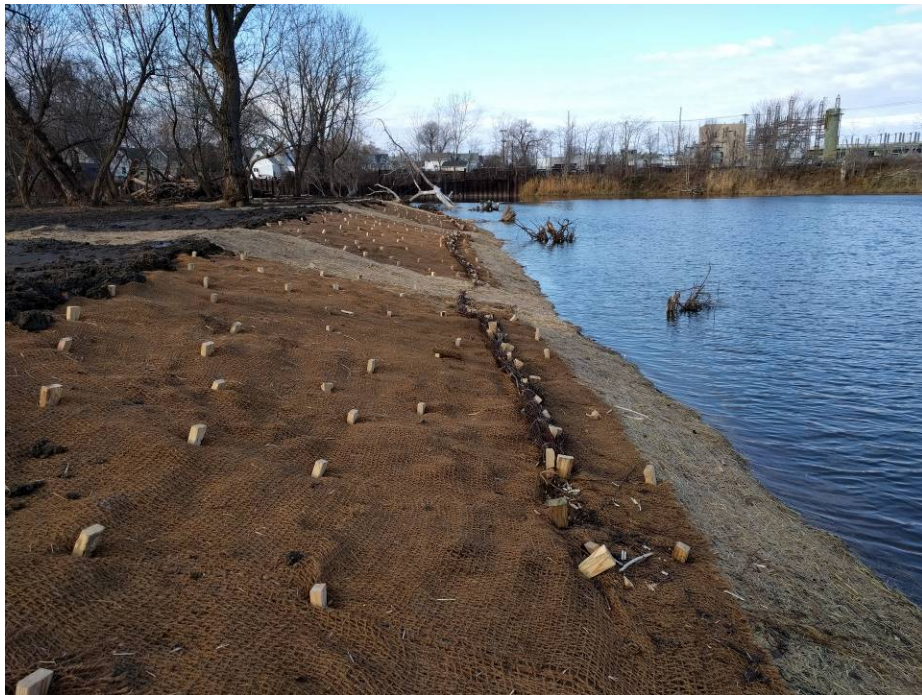
Photo 19. Reach 3. Looking downstream; 08 December 2016. Fiber matting, hay compost roll, and live fascines shown on cutback slope.
