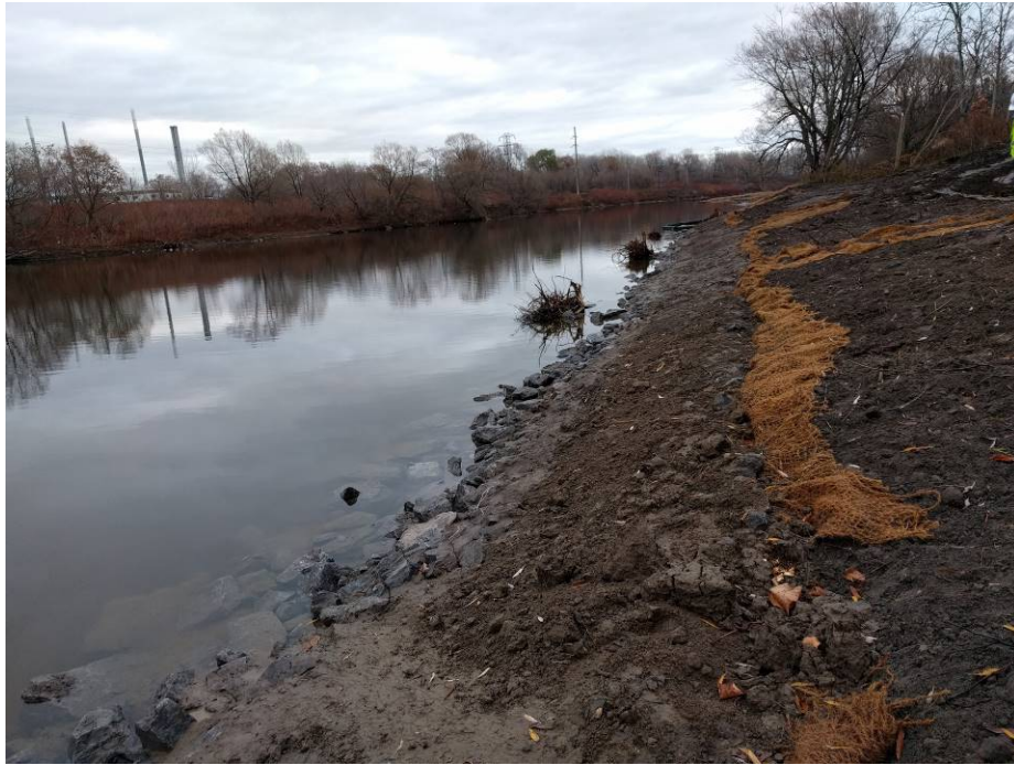
Photo 16. Reach 3a. Looking upstream; 30 November 2016. Toe protection and rootwads shown near river edge.
