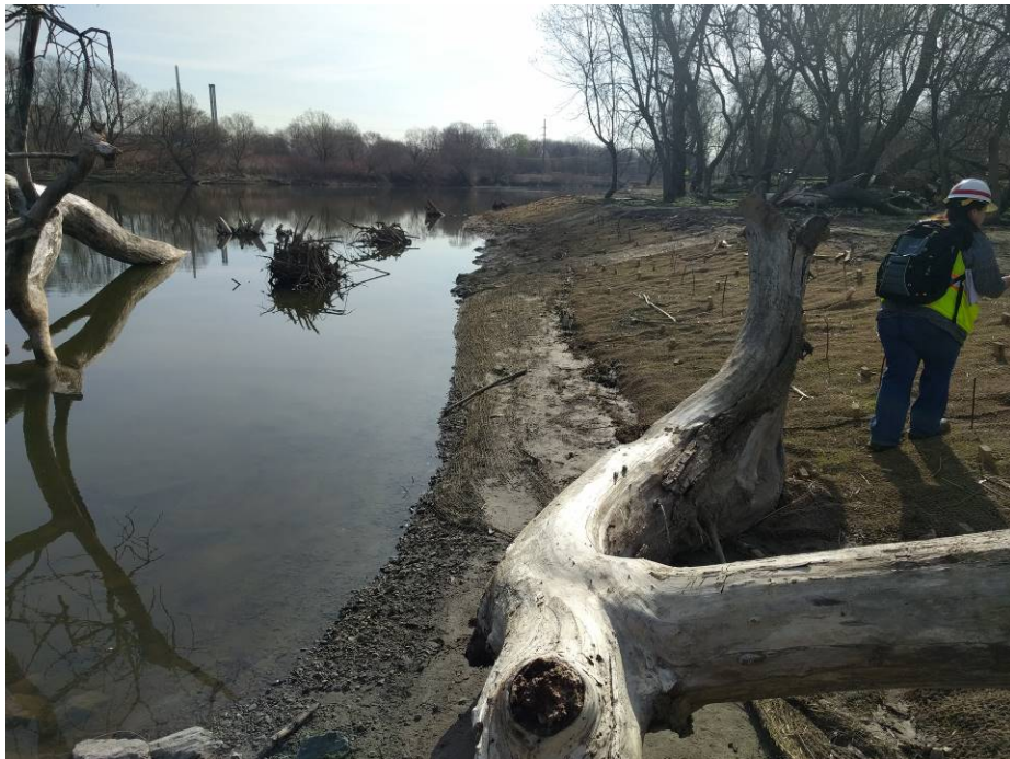
Photo 21. Reach 3. Looking upstream; 13 April 2017. Rootwads seen in river edge areas. Livestakes installed on cutback slope.
