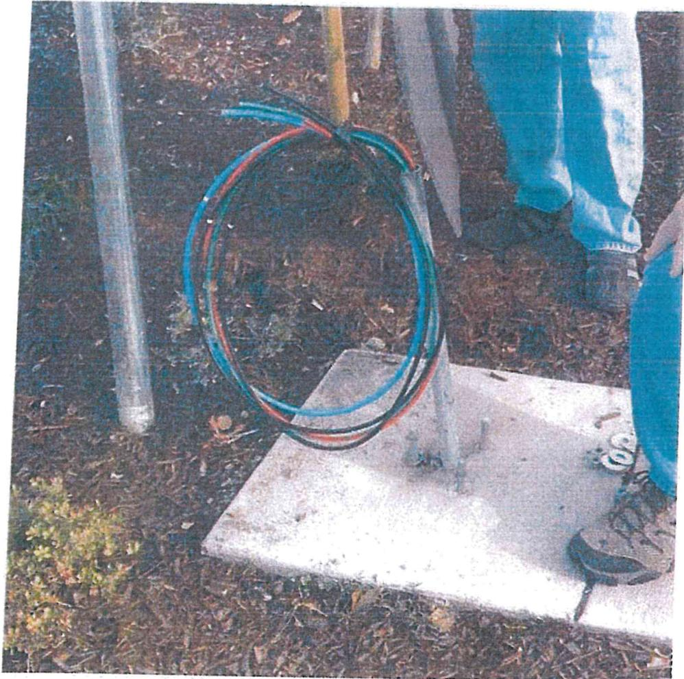
(Proper concrete pad with anchor bolts and conduit stub-up)
