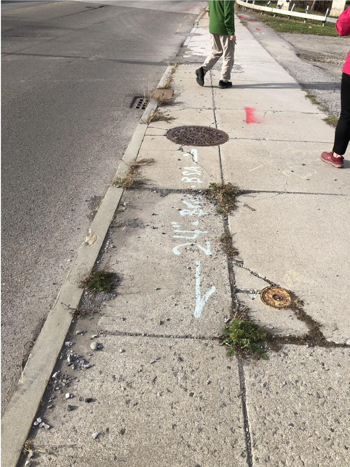
Photo 6: Looking west along Seneca Street at utilities located beneath sidewalk. An existing gas line, 24" brick combined sewer, 12" PVC separate storm drain system, and electrical lines all run underground along Seneca Street.
