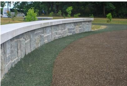
The multi-use pathways around the parking lot will consist of 5,350 SF of flexi-pave pavement, which has proven to be a reliable permeable pavement material and is ADA compliant. Flexi-pave is composed of recycled vehicle tires and removes up to 90% of soluble phosphates and nitrates. The appearance of the pathway will incorporate both naturalized colors and the Buffalo Blueway colors with a distinctive design unique to the Park.
