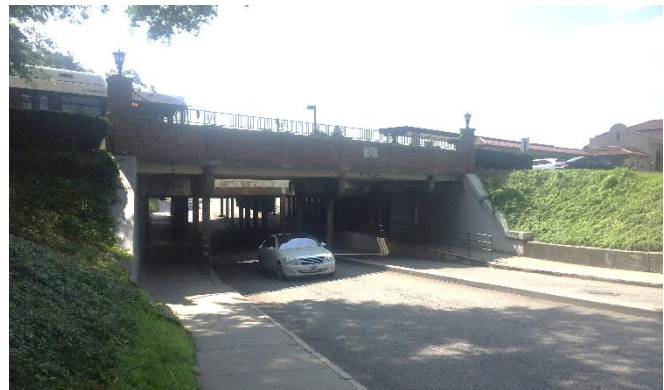
Bronxville's Metro North Underpass
