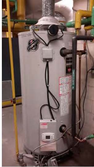
Figure 10: 80-gallon Bradford White DHW Tank
