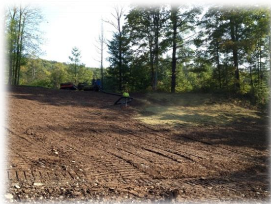
Figure 6: Prior to planting the hillslope, top soil was imported and spread to allow for improved planting medium. September 2013.
