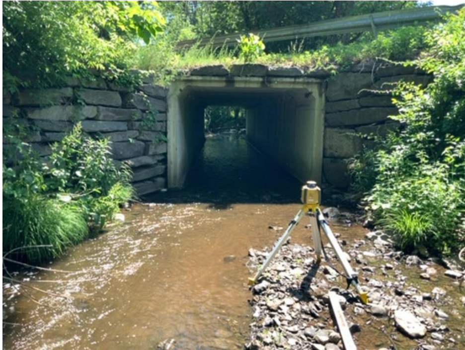
An example of headwalls and wingwalls on Hurley Mountain Road. Source: Ulster County Department of Environment.
