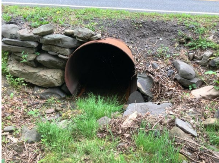
An example of a deteriorating embankment on Kripple Bush Davis Corners Road. Source: Ulster County Department of Environment.
