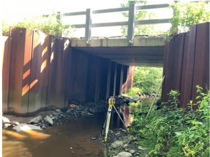
An example of abutments. Source: Ulster County Department of Environment.
