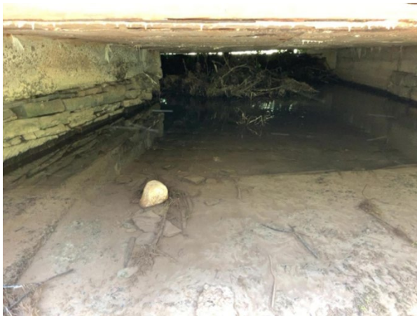
An example of a clogged crossing. Source: Ulster County Department of Environment.
