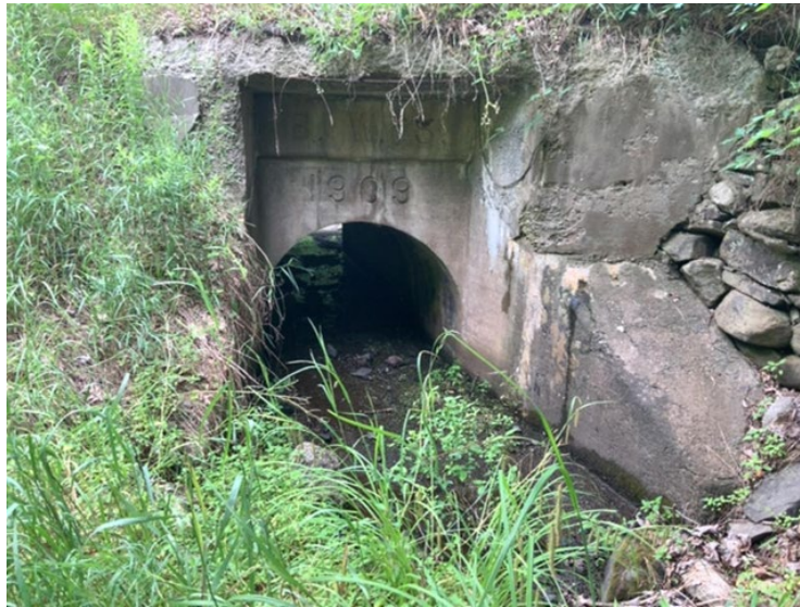
An example of a crossing that is aging on Atwood Road. Source: Ulster County Department of Environment.
