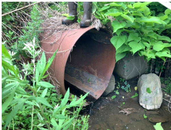
An example of a crossing that lacks natural substrate on Atwood Road. Source: Ulster County Department of Environment.
