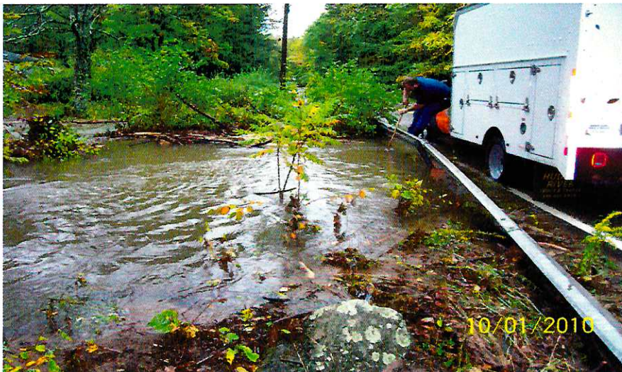
Figure 4: Ulster County Staff Attempting to Unclog the Inlet of the Mine Hollow Culvert
