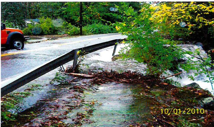
Figure 5: Watson Hollow Road Flooding due to Blockage at the Inlet of the Mine Hollow Culvert
