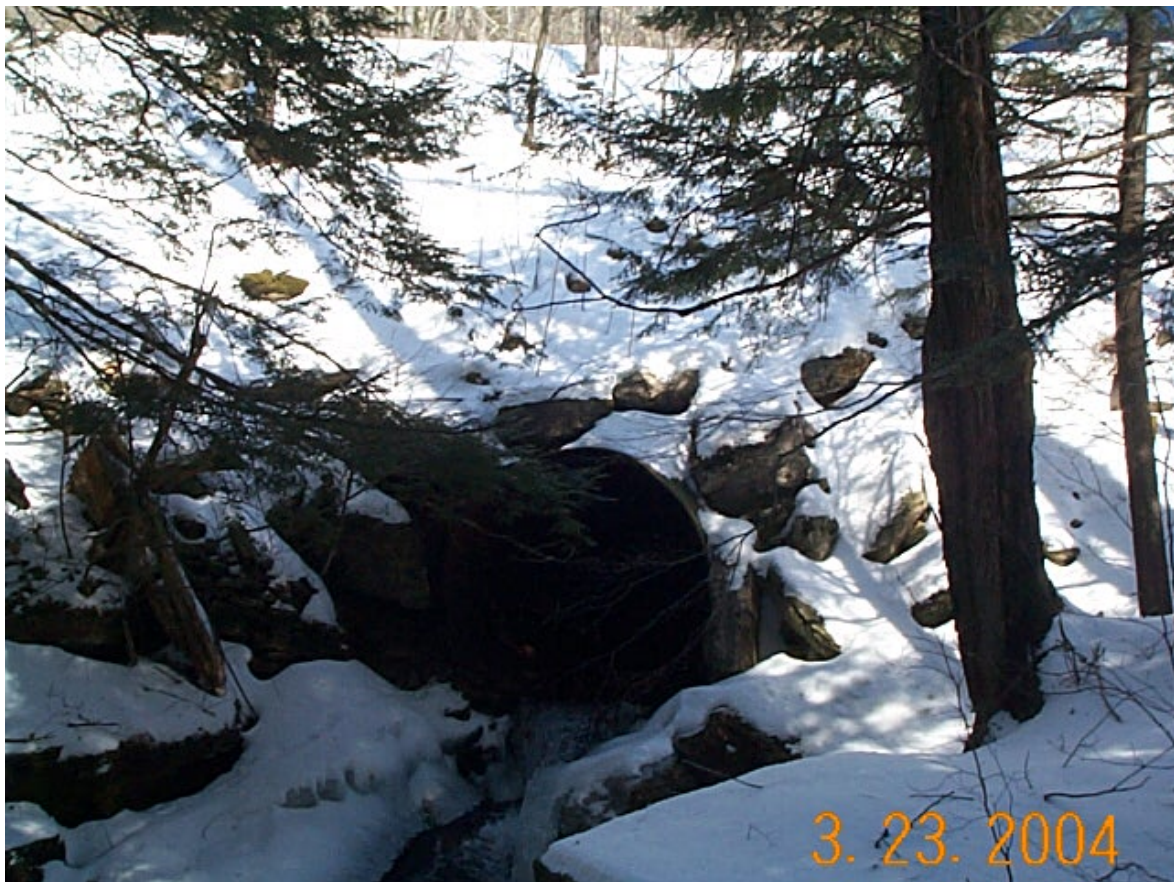
Photo 1. Eight foot diameter pipe outlet prior to Fisher Bridge construction
