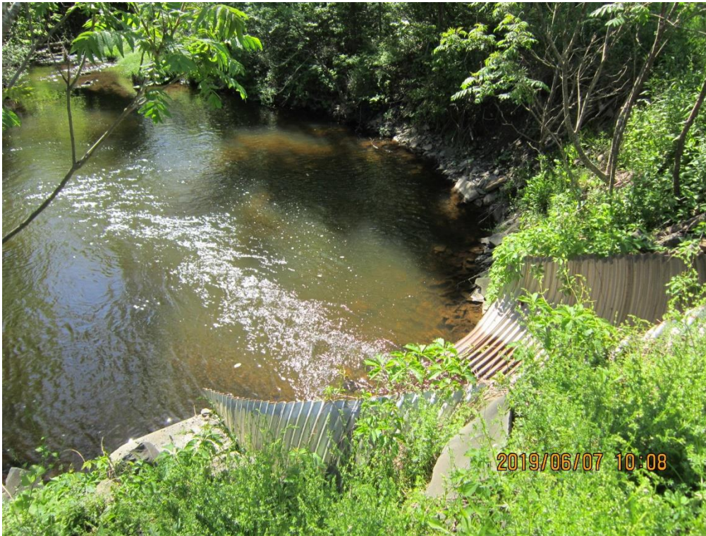
Photo 3: View looking southeast at outlet of Culvert – from edge of highway.
