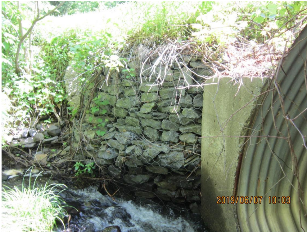
Photo 7: Gabion wall at left side of inlet of Culvert – looking northeast.
