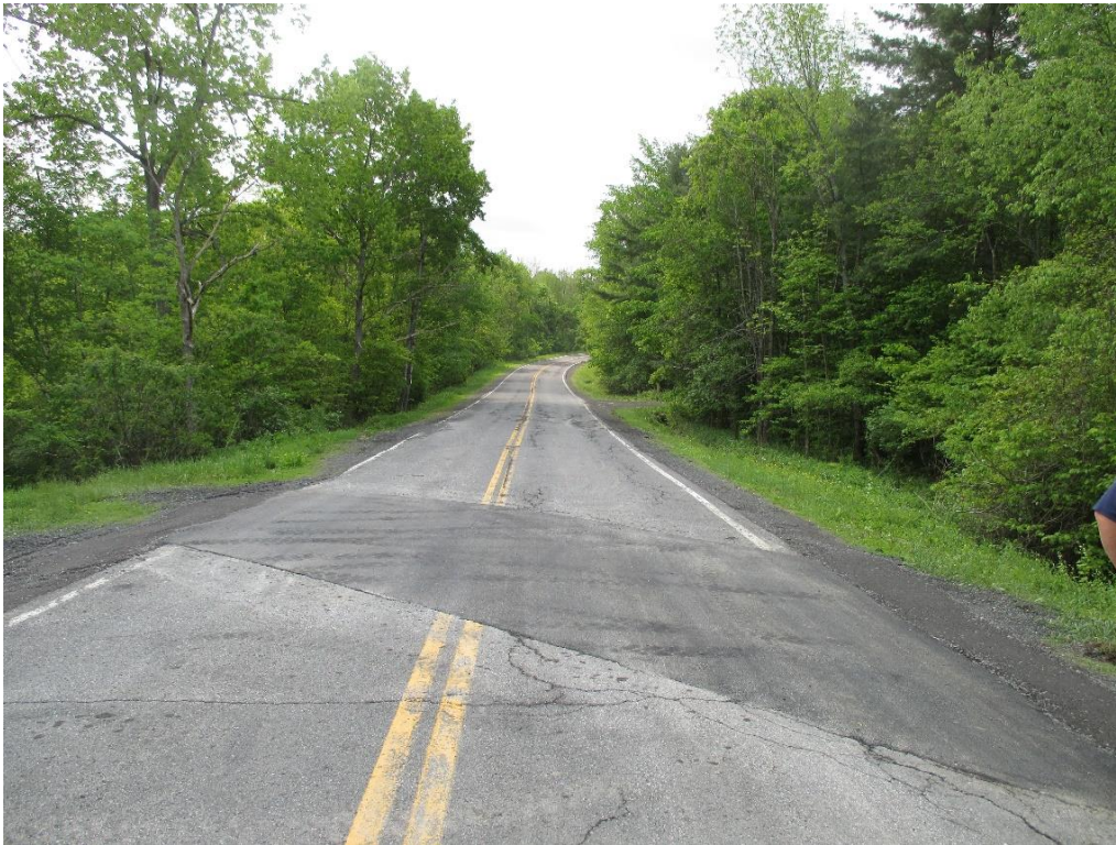
Photo 9: Asphalt patch over Culvert – looking south.
