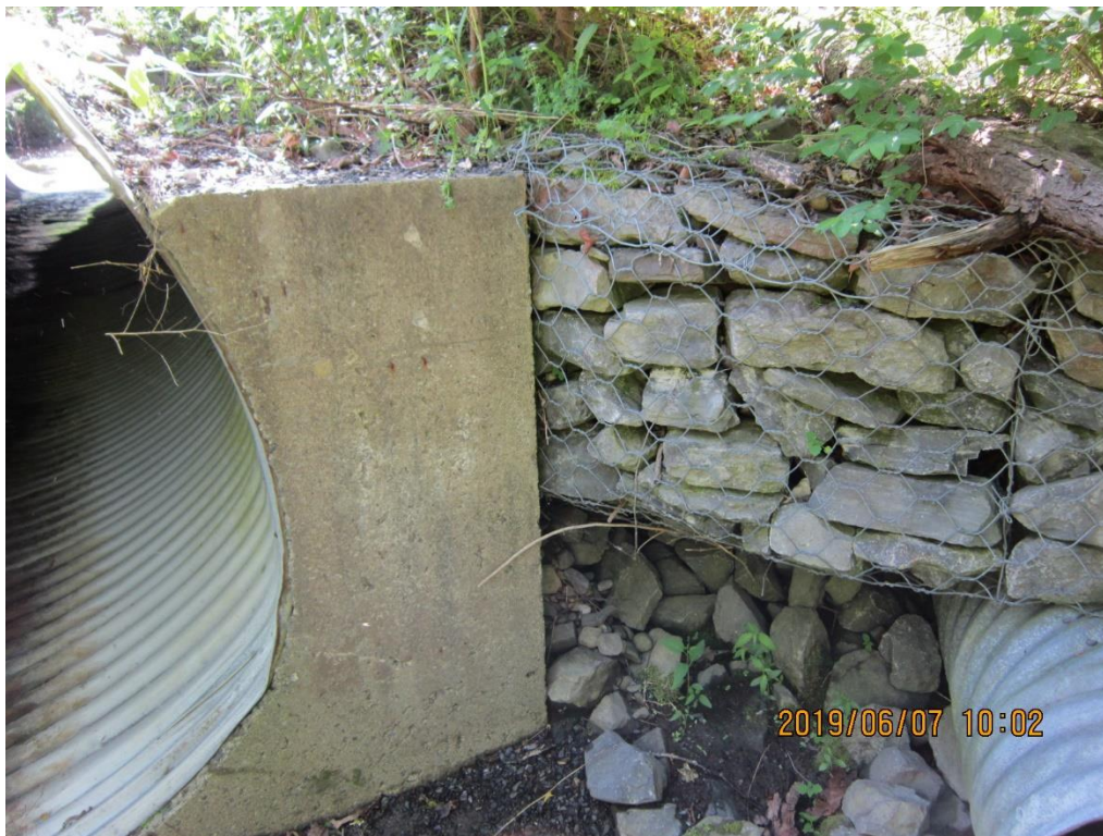
Photo 8: Gabion wall at right side of inlet of Culvert – looking southeast.
