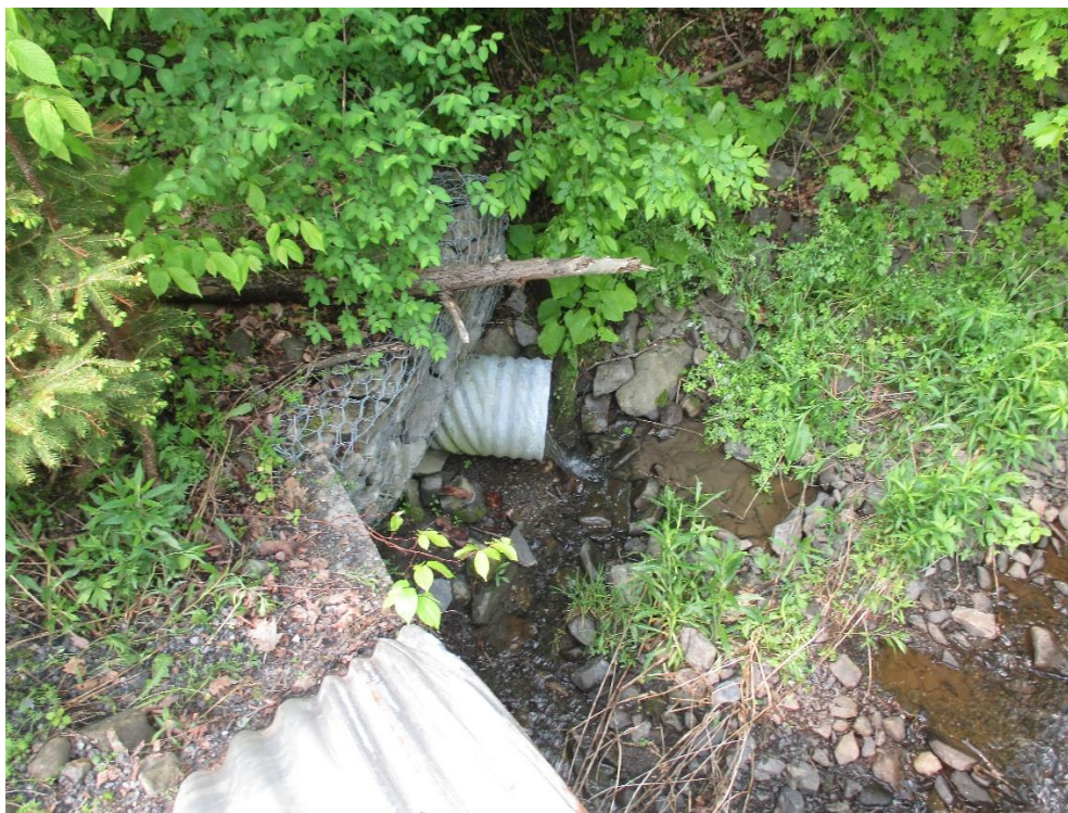
Photo 6: Drain pipe in southwest corner of inlet of Culvert.
