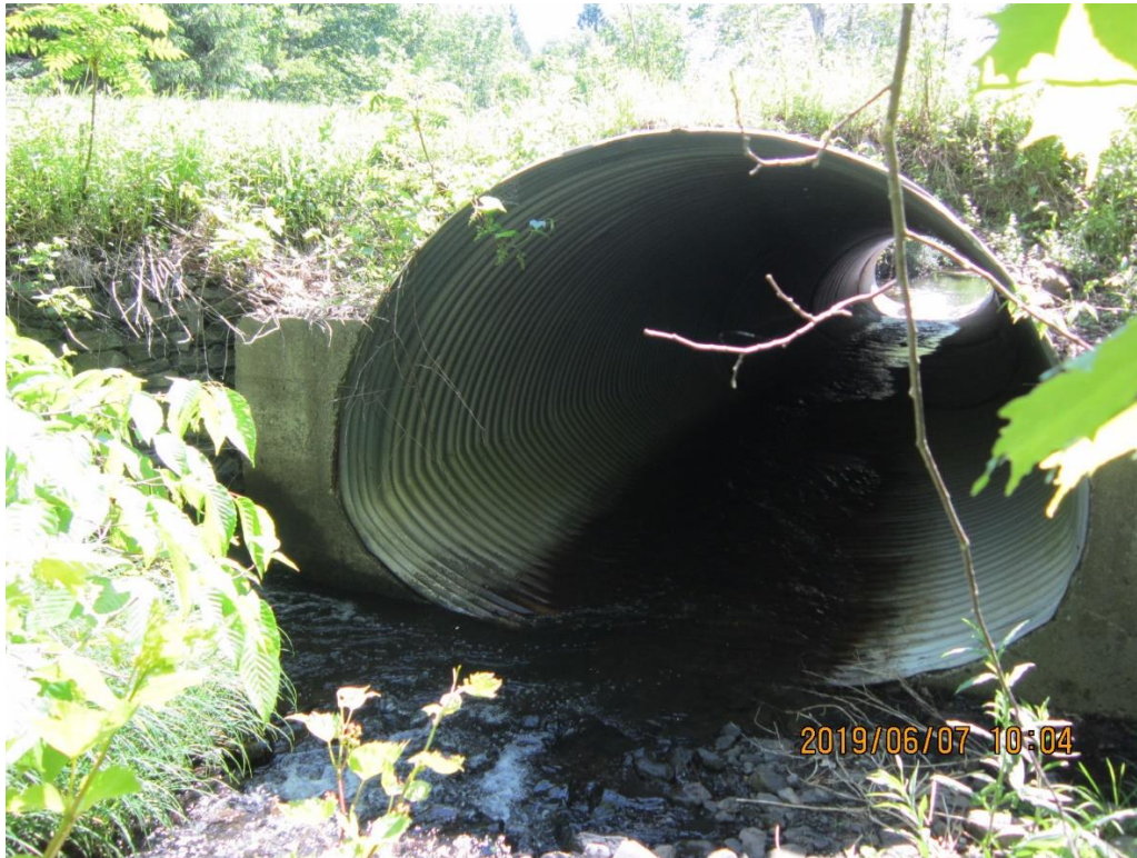
Photo 5: Inlet of Culvert – looking east.
