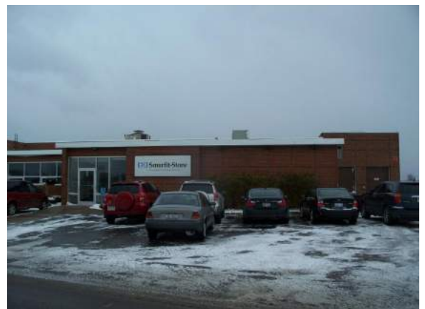
View of main office from Robinson Street
