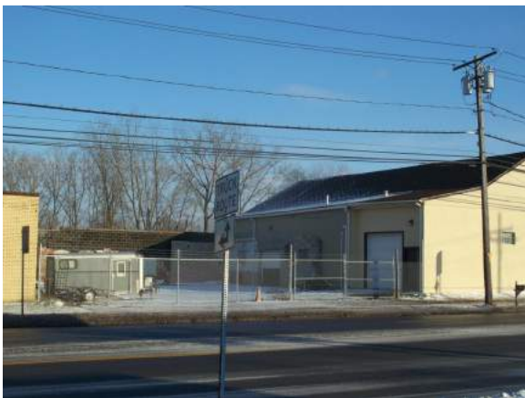
View of Building from River Road.
