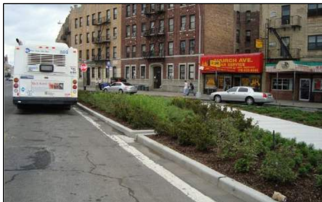
The narrowing of a roadway is an excellent opportunity to provide green infrastructure improvements to enhance the function and aesthetics of the neighborhood.
