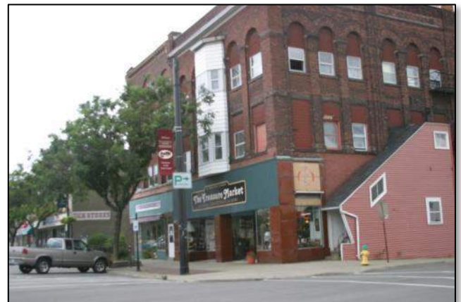
The 'Teddy Bear' building, shown here prior to renovations, is located within the Downtown Central Business District.
