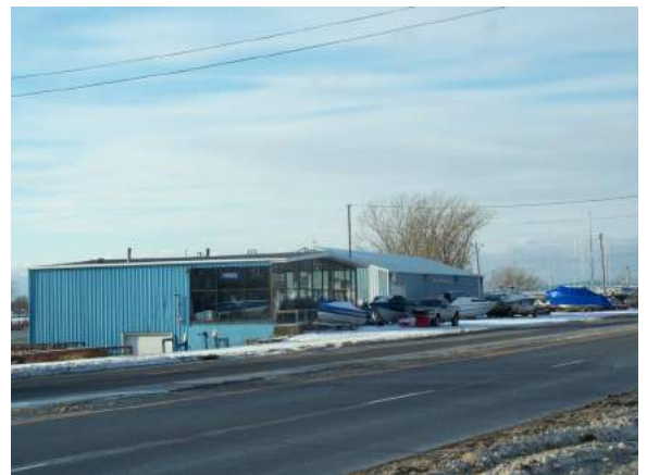
View looking northwest
