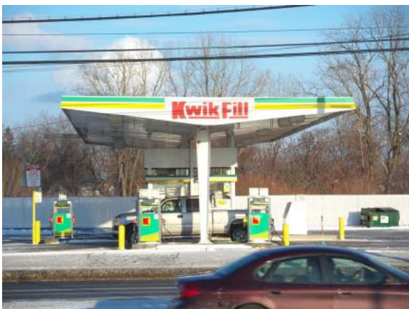
Close up of site
