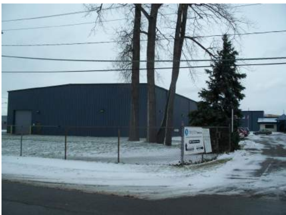
View looking north
