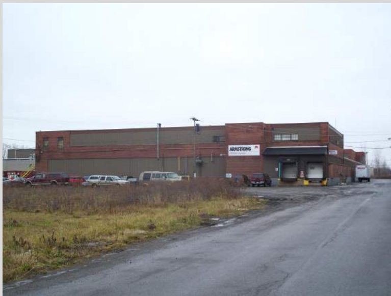
View from East and Oliver
