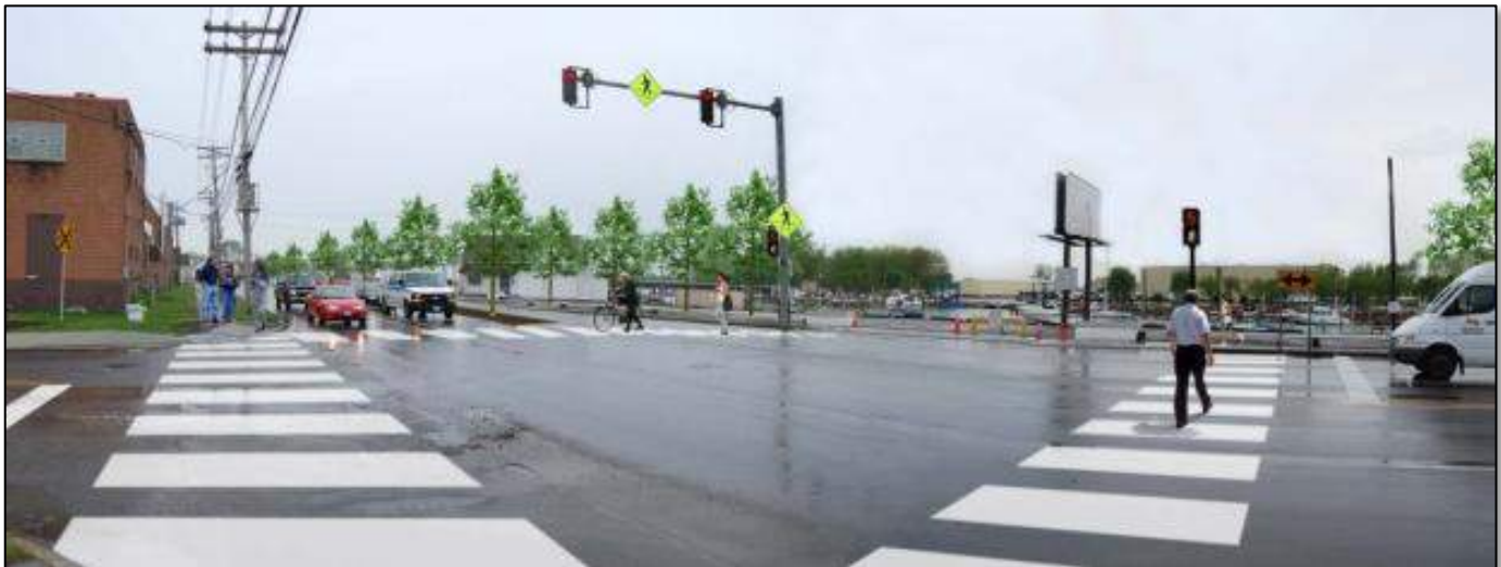
Figure 8: View of River Road with proposed enhanced crosswalks, street trees, and a central median where possible to reduce the overall scale and impact of the roadway corridor.
