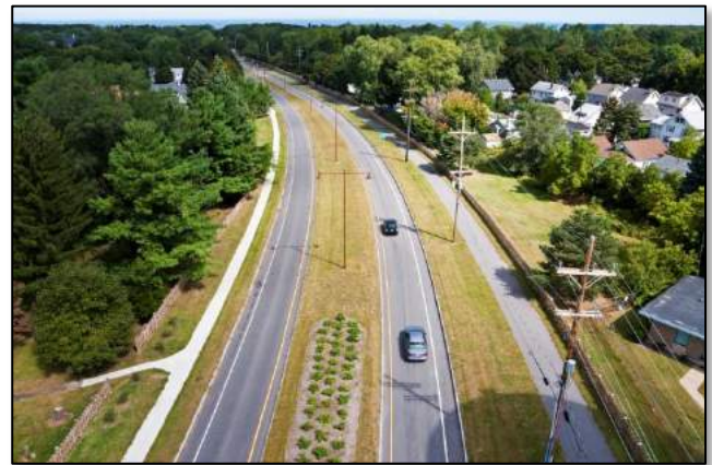
Seabreeze Drive was significantly reduced in roadway cross section, and included sidewalks, a multiuse trail, and a central median.
