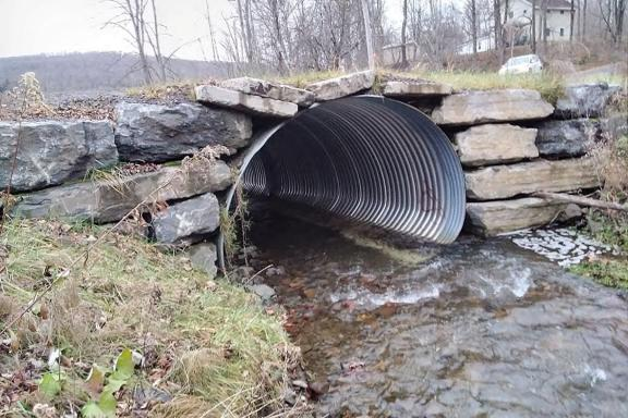
It can be shown, that the huge Edwards Road culvert replacement project done in coordination with FEMA and approved by the Army Corps of Engineers, abides by the CRRA regulations shown on page 39 of the CRRA Flood Risk Management Document. The required additional two feet of roadway freeboard above the projected checkflow was included in the authorization.
