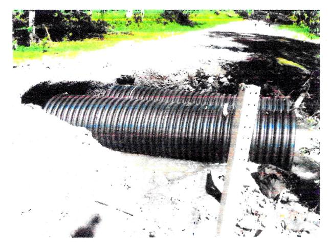
This is the Height of The (a) 4 Foot Tubes The Town will RAISE The BARdway By 24" TO 30" To fit The Rise of New Titol. Est of Roadway To Be Raised will Be 150 To 180 Feet, with a base of shahe, Top with Item 4 gravel
