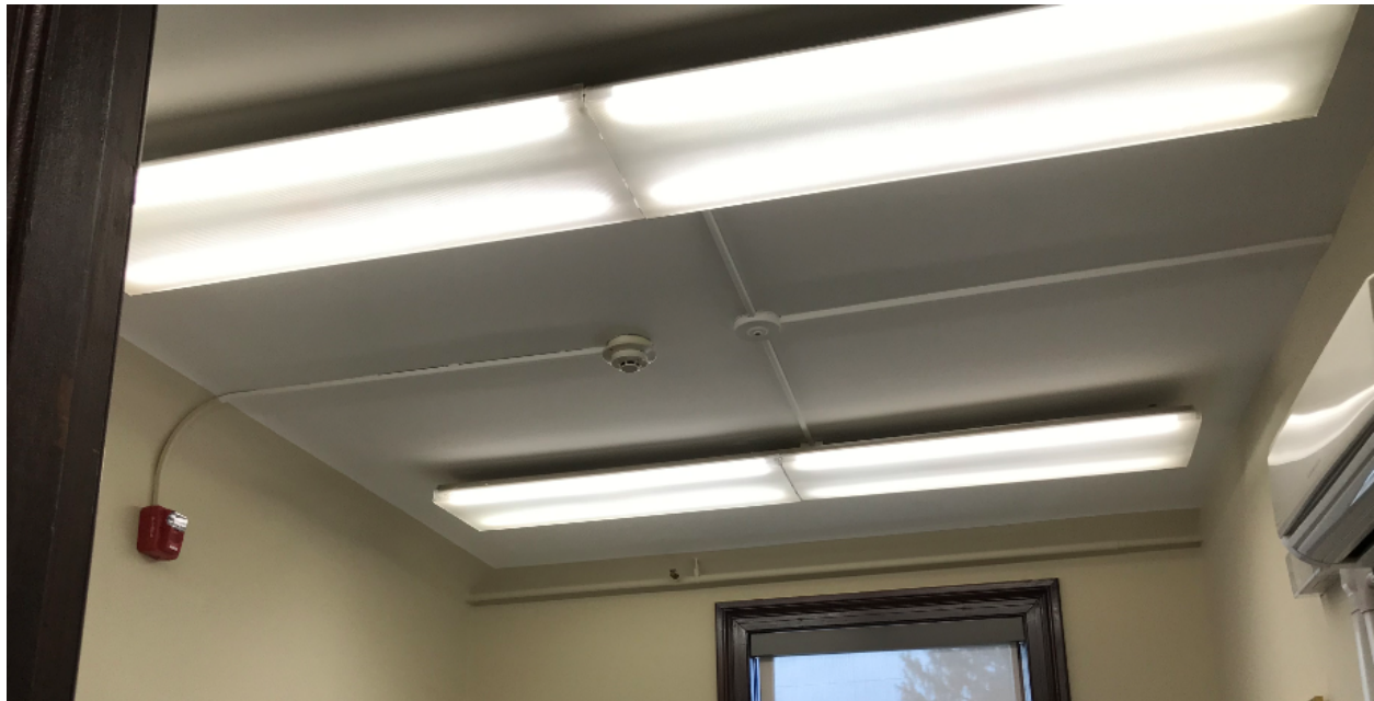
Photo 16: Typical T8 LED Fixtures
