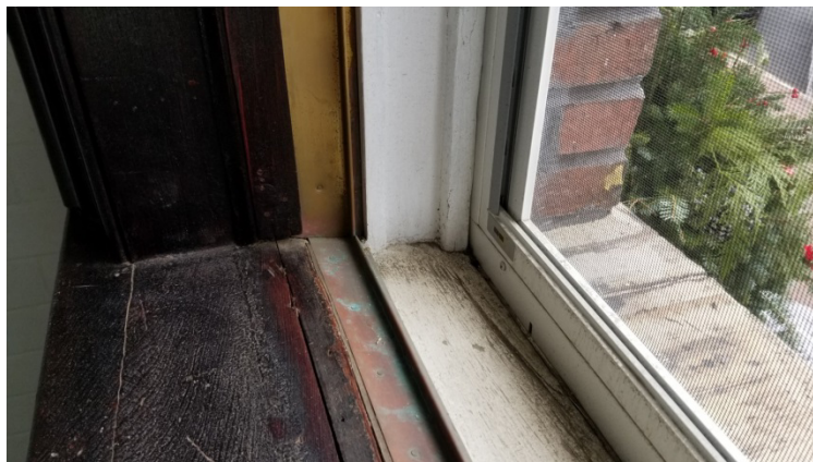
Photo 9: Typical Original Window with Storm Window
