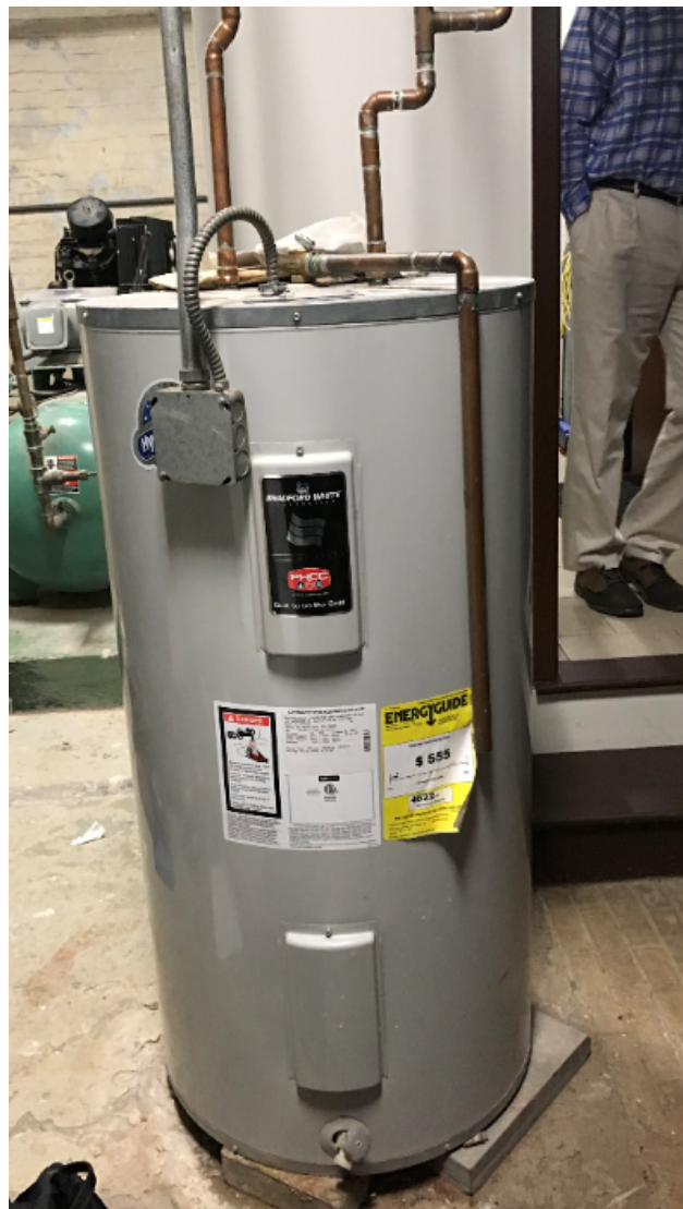
Photo 7: Storage Hot Water Heater
