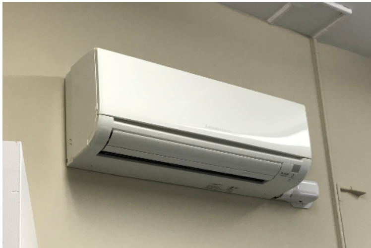
Photo 5: Typical Indoor Evaporator
