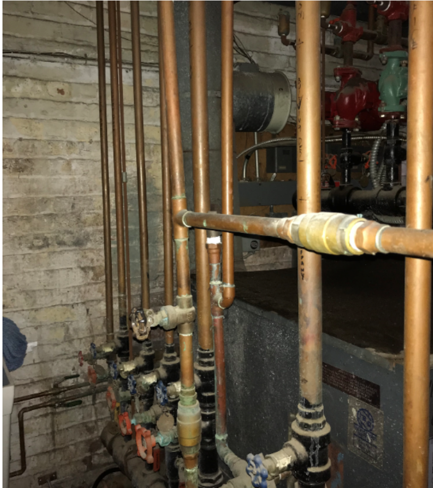
Photo 2: Uninsulated Hot Water Piping
