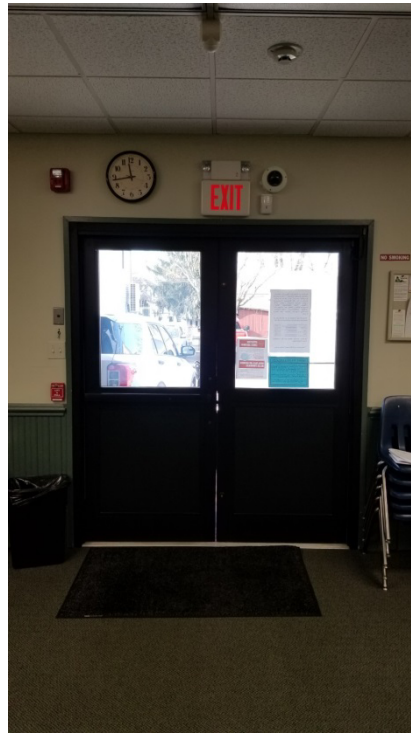
Photo 11: View of Village Court Doors. Note daylight at lock, bottom and meeting of doors.
