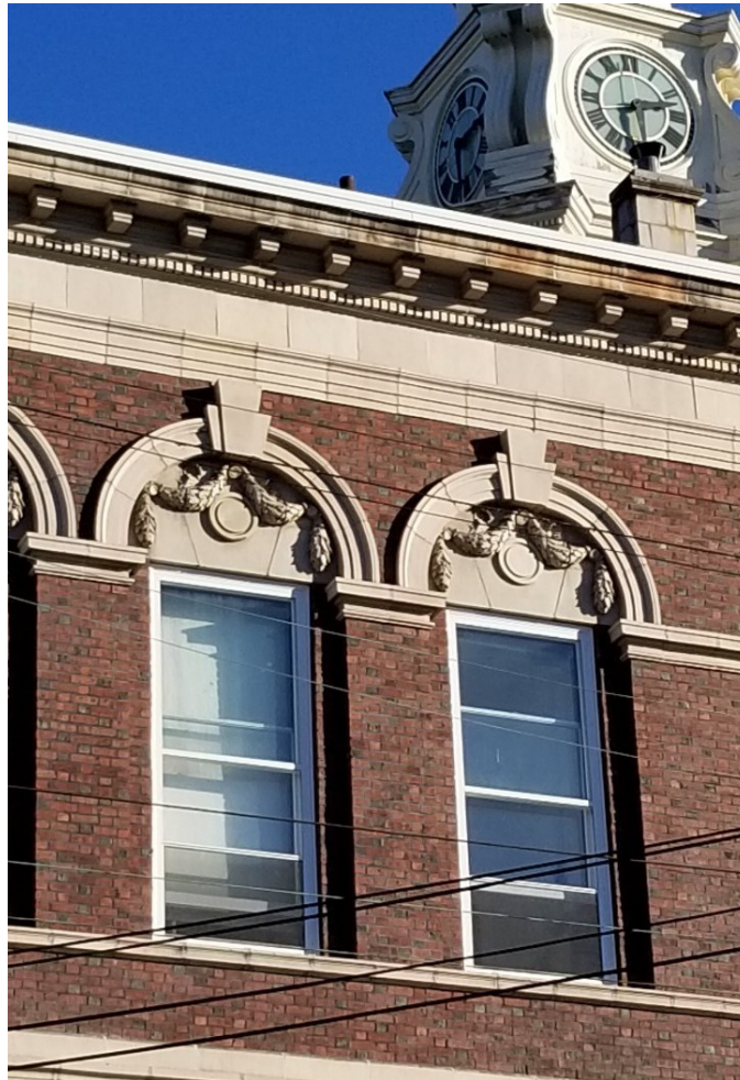
Photo 10: View of Exterior Showing Storm Window. The 2 nd Floor original sash appears to be open
