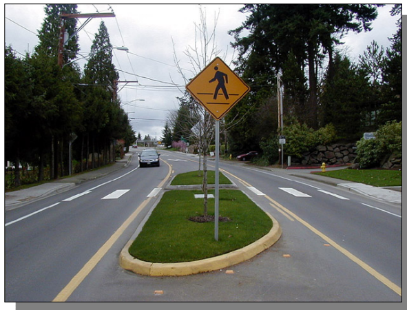
Simple engineering measures such as pedestrian refuges can improve real and perceived safety.
