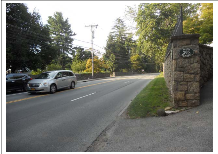
Existing conditions on the east side of Broadway will make inclusion of sidewalks problematic given lack of available right-of-way, topography and physical impediments.
