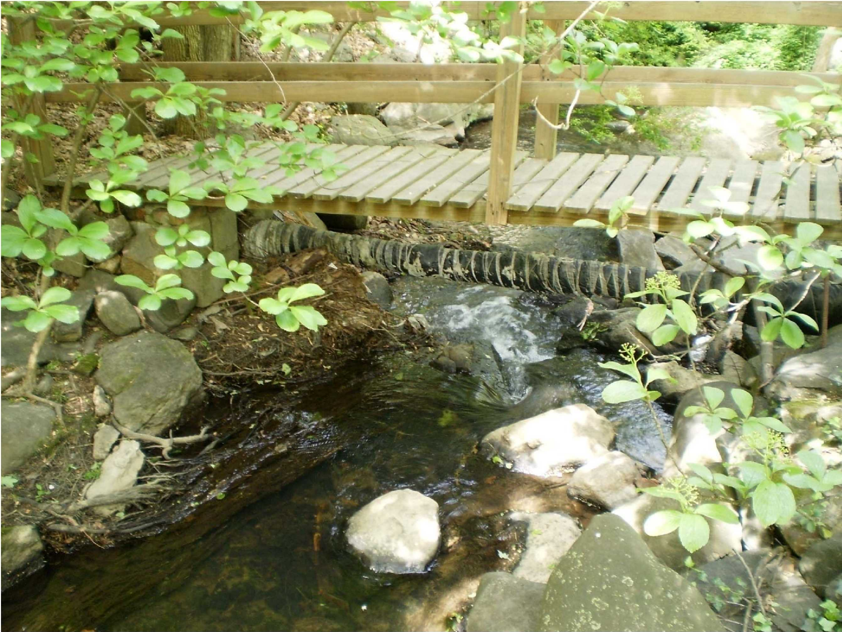
Sewer service and walkway impedes flow.
