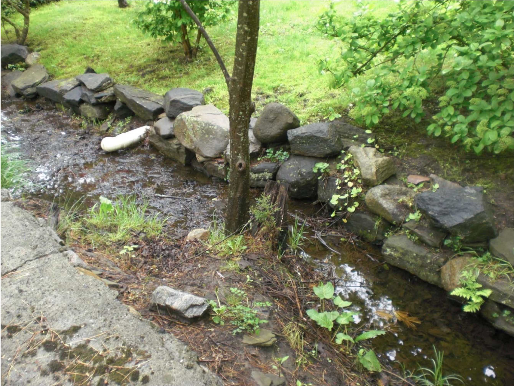
Sediment Buildup, Vegetation, and channel failure
