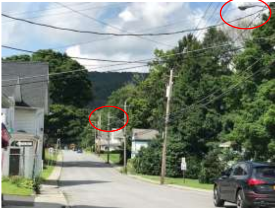
Mill St., Dover Plains street lights before upgrade
