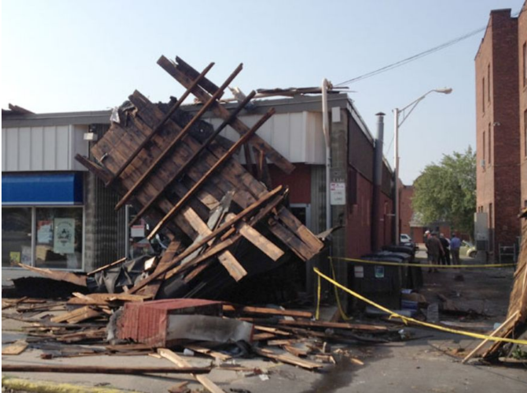
Figure 11 : Damage from the 2012 Microburst Storm
