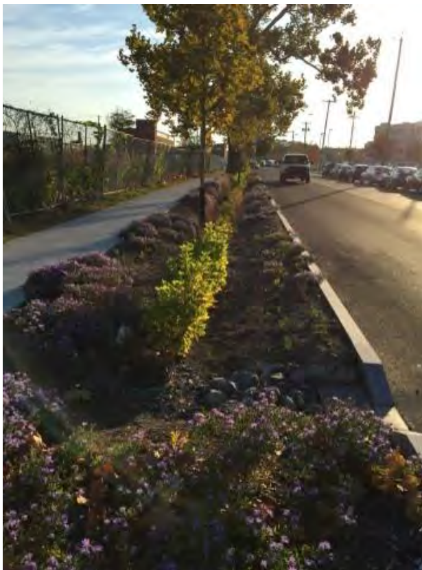
Figure 1. Bioretention area capturing runoff from street in Syracuse, NY. Credit: NYS Environmental Facilities Corporation.
