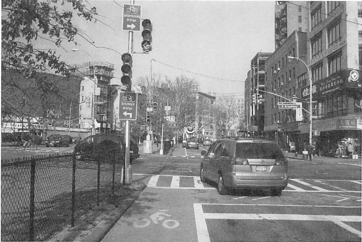
Figure 53 Example of Bike Signals at an Intersection
