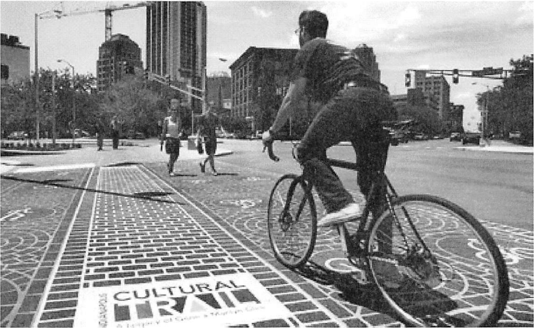
Figure 56 Intersection with Pavers to Help Designate An Intersection as a Mixing Zone
