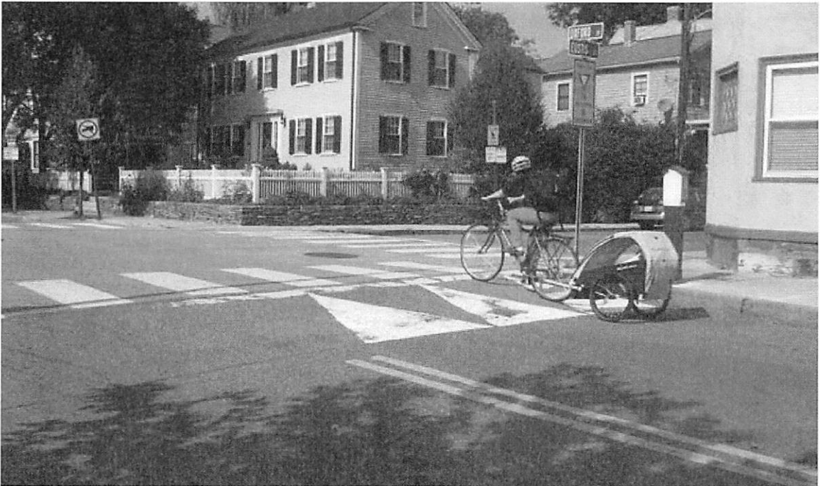
Figure 54 Raise Intersection and Bike Crossing
