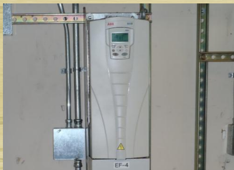
VFD for Air Handler Unit
