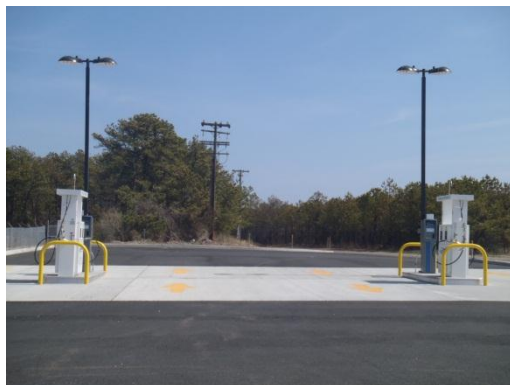
Two Fast-Fill CNG Dispensing Islands
