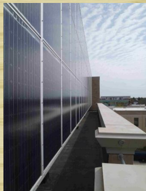
24 kW South Facing, Two-Sided, Solar Panel Array
