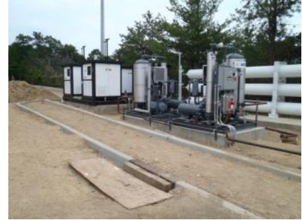
Installation of Compressors, Dryers, and Storage
