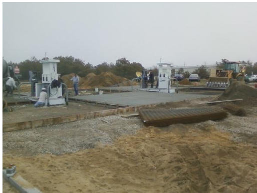
Workers Installing Dispensing Islands
