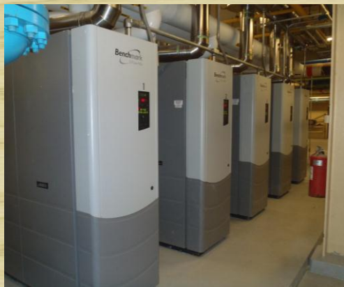
Condensing Boilers
