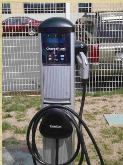
Charge Point Level I&II Electric Vehicle (EV) Charging Station
