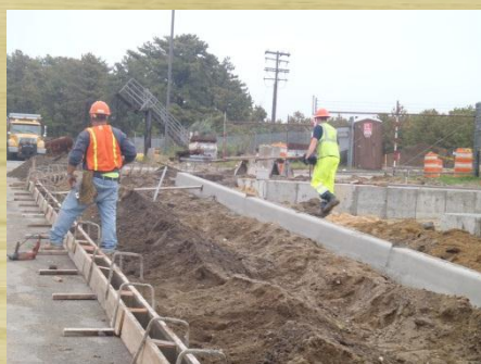
Workers Casting a Concrete Curb
