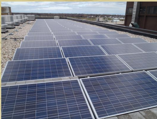
24-KW PV System Array
