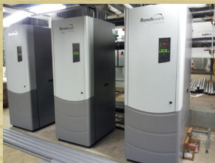
Three AERCO Benchmark 1.5 Condensing Boilers Installed at the County Center
