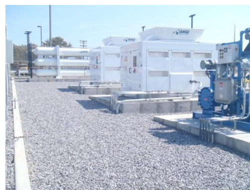
Compressors, Dryers, and Storage Equipment
