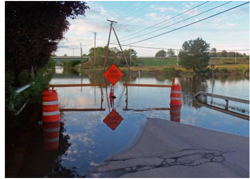
NY 416 flooded by Wallkill River after Lee. (Photo courtesy of Daniel Case)
