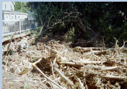
Debris and Road Collapse in the Village of Ellenville (Photo courtesy of NYRCR Ulster Plan)
