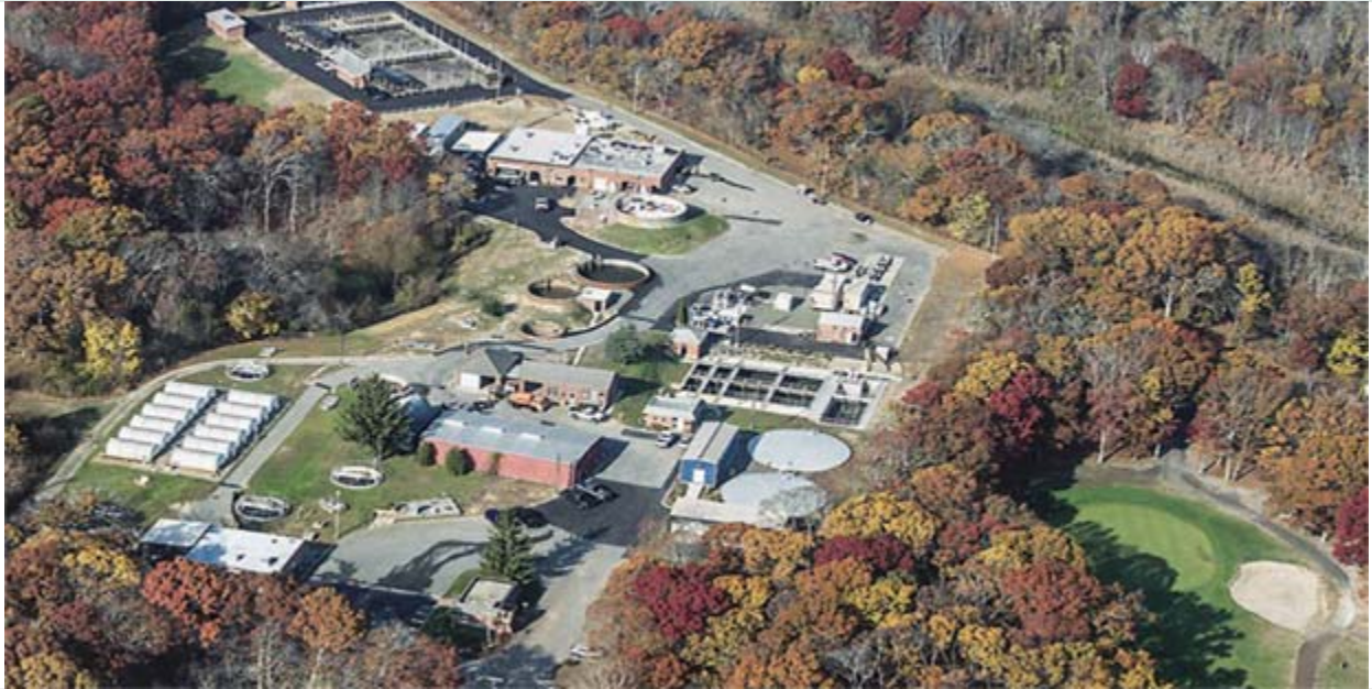
Aerial view of the upgraded Riverhead sewage treatment plant and the adjacent Indian Island Golf Course.
