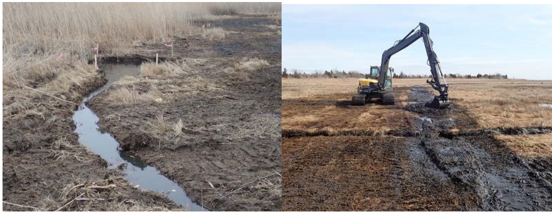
Left: Runnels. Right: Filling Ditches:
