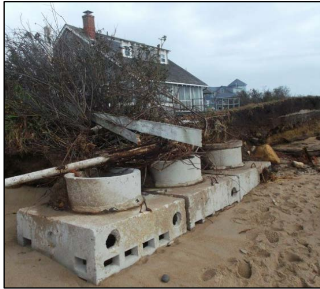
Septic systems uncovered during a coastal storm 108 .
