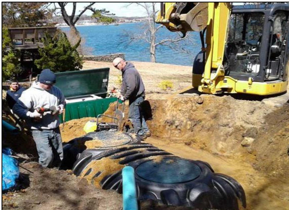
Installation of an I/A OWTS in Suffolk. Photo courtesy of Suffolk County.
