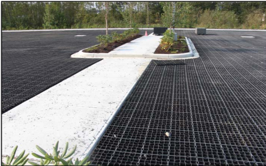
Parking lot constructed using permeable pavement. 182
