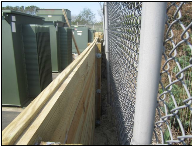
Captree and Ocean Beach flood walls. Photos courtesy of PSEG-LI.
