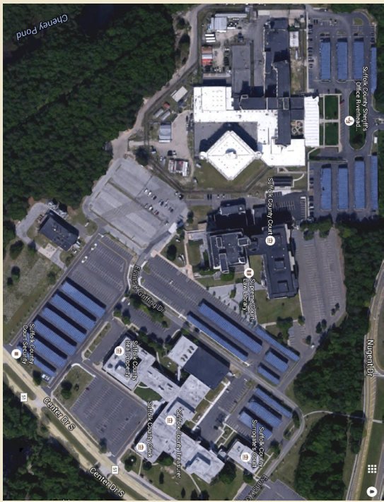
Aerial view of solar carparks at Suffolk County Riverhead Complex
