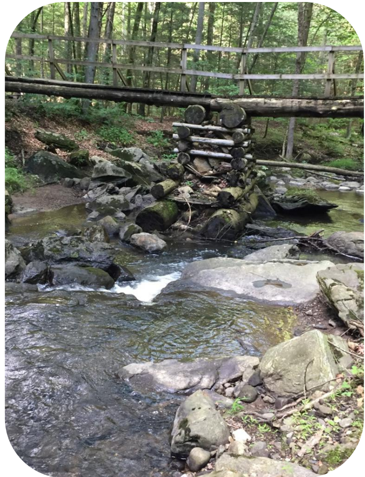
Appalachian Trail bridge over Deuel Hollow Brook.
