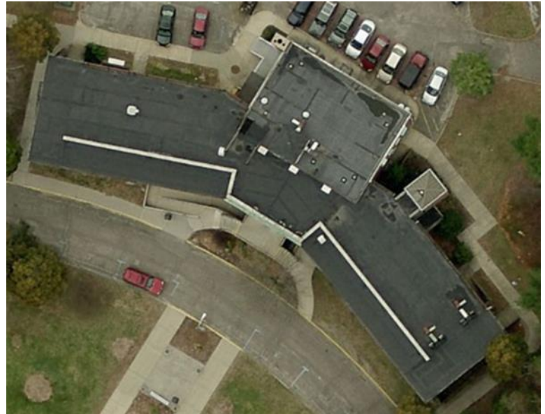
Figure 10: Roof of Kreiling Hall.
