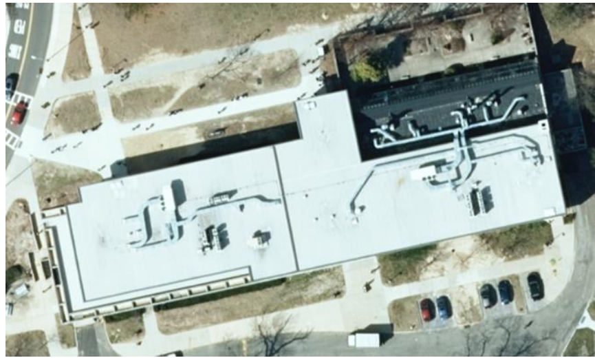
Figure 16: Roof of Southampton Building.
