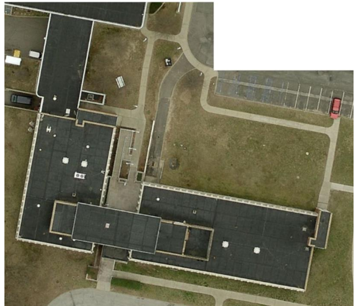
Figure 23: Roof of District Attorney Roof.
