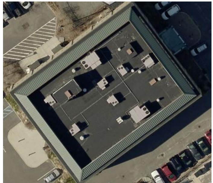
Figure 37: Roof of Cornell Coop. Ext.
