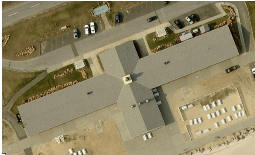
Figure 38: Roof of Pavillion.
