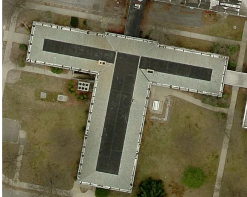
Figure 25: Roof of Labor Department.
