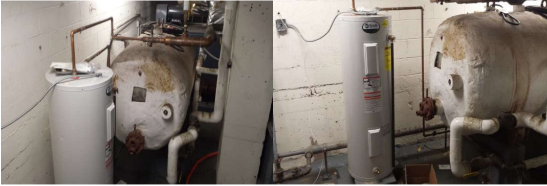
Photos above show existing electric water heater and steam to hot water heat exchanger
