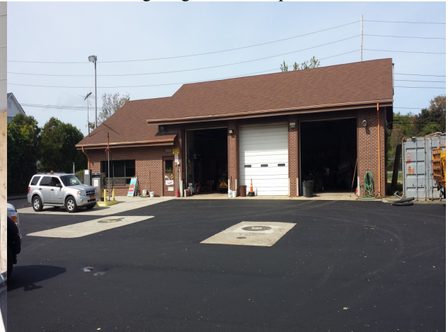
Shown above are three exterior wall pack fixtures
