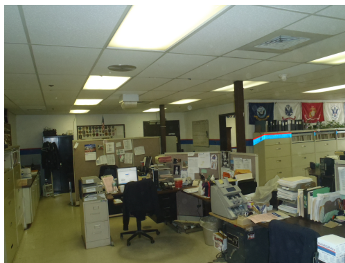
Shown above is the office area illuminated with 2 x 4 lay-in fixtures
