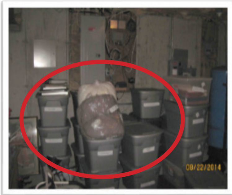
Photo D3: Working clearance not maintained: NEC 110.26
