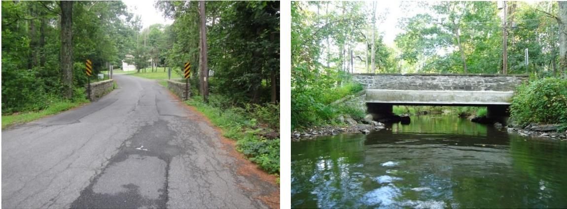
**Figure 1. Photographs of the downstream Aspinwall Road Bridge. The relatively narrow bridge opening and limited vertical clearance constrict streamflow during high flow conditions.**
