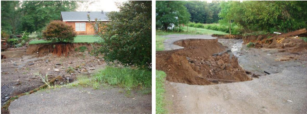
**Figure 2. Photographs of erosion caused by the overtopping of the left abutment at the Mill Road dam during Tropical Storm Irene in 2011**
